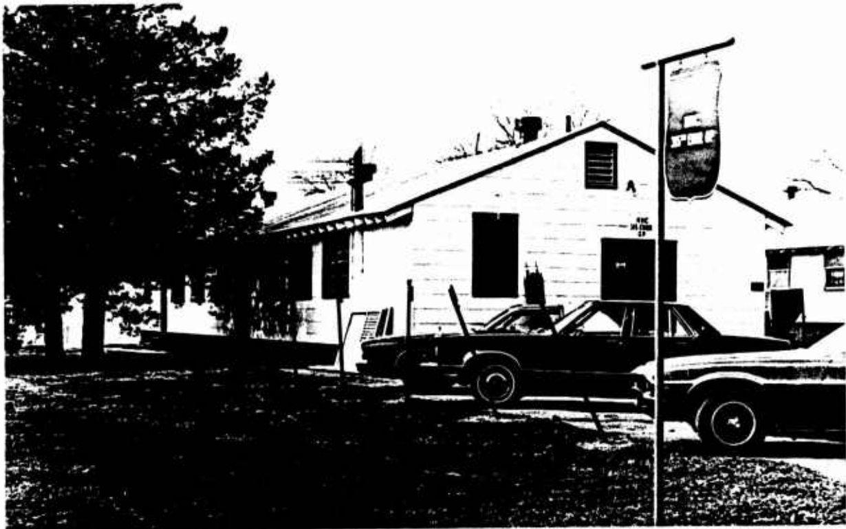
Illustration 10 View of Building 269. This one-story building housed the Reception Center's administrative offices. (Source: Field inventory photograph, 1984, Barbara Hightower, Building Technology, Inc.)
