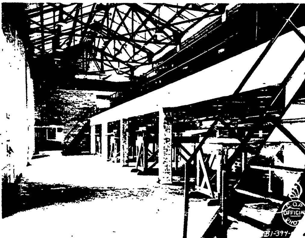
Figure 7: Exterior and interior views of Ammonium Nitrate Crystallizer Building (Building N-5), showing concrete frame, steel roof framing, and structural clay tile infill. Cornhusker Ordnance Plant Official Photos, U.S. Army Corps of Engineers, February, 1944. (Source: AMCCOM Historical Office, Rock Island Arsenal)
