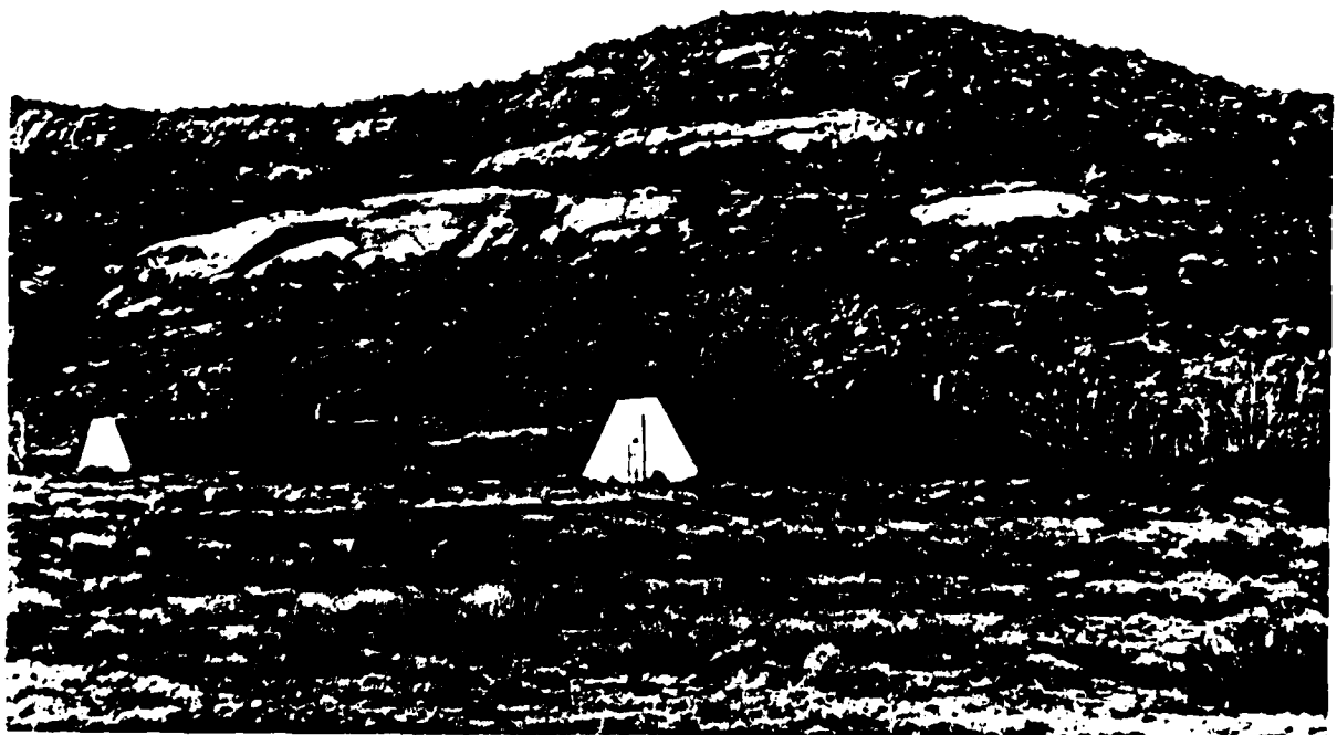
Illustration 4 View of Igloos C1101 and C1102 and Storage Pad Y1101. Between May and September 1941, 650 standard ammunition storage igloos were built at the depot. Storage facilities were later expanded with the construction of 303 "Y" type open storage pads such as Y1101, most of which were placed between the existing igloos. (Source: Field inventory photograph, 1984, Barbara Hightower, Building Technology, Inc.)
