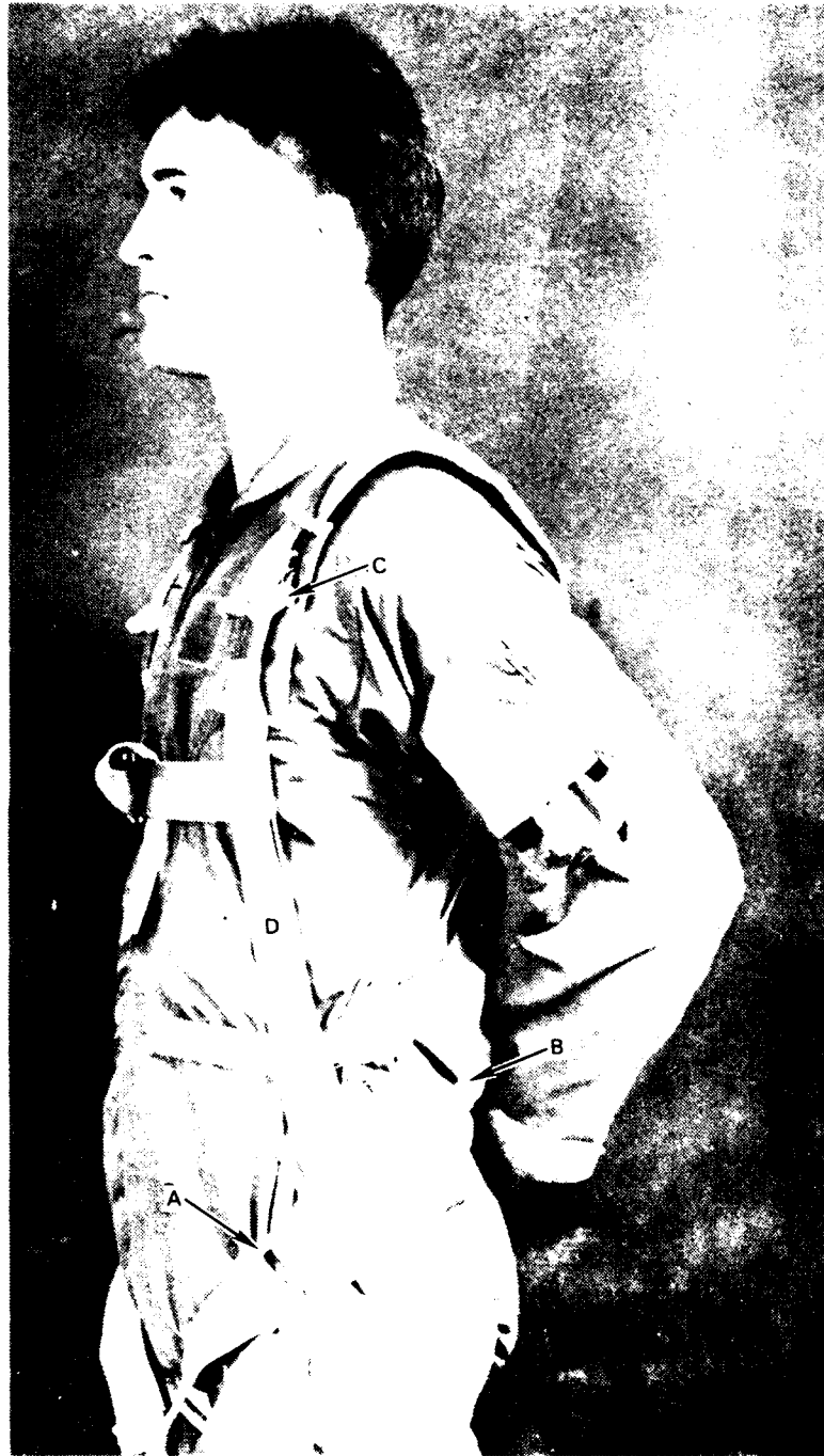
FIGURE B-3. Side View of Trainee in Harness. Harness is constructed from MIL-W-4088H Type 7 webbing. (A) Leg strap adjuster is MS-22040-1; (B) solid link in diagonal back strap is MS-70108; (C) connector links are MS-22021; (D) main lift web is 20 inches from bottom of leg strap junction to top of load loop. Exact dimensions are not critical as long as harness is symmetrical and fits the trainee properly.
