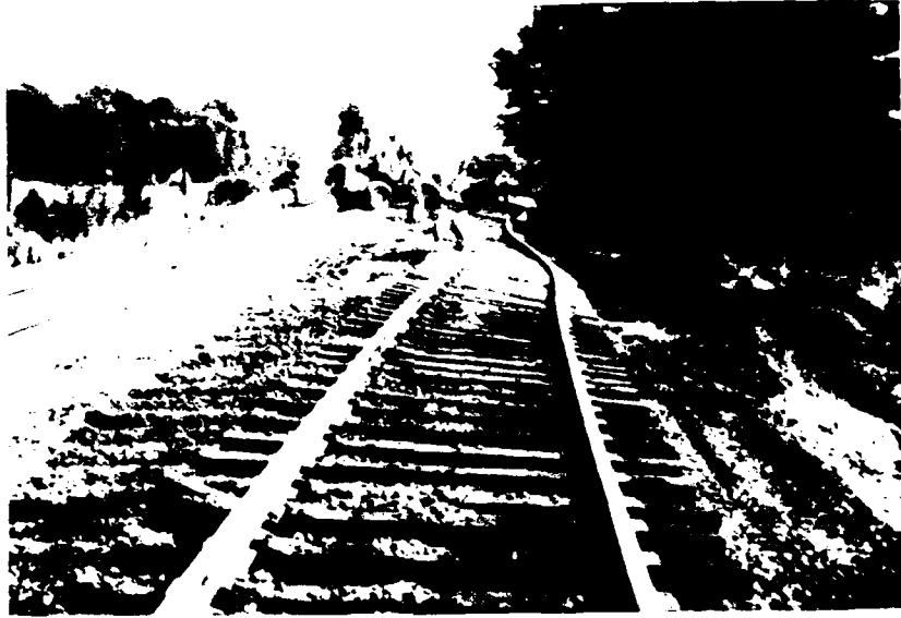
Figure 63. Moving track to side for construction
