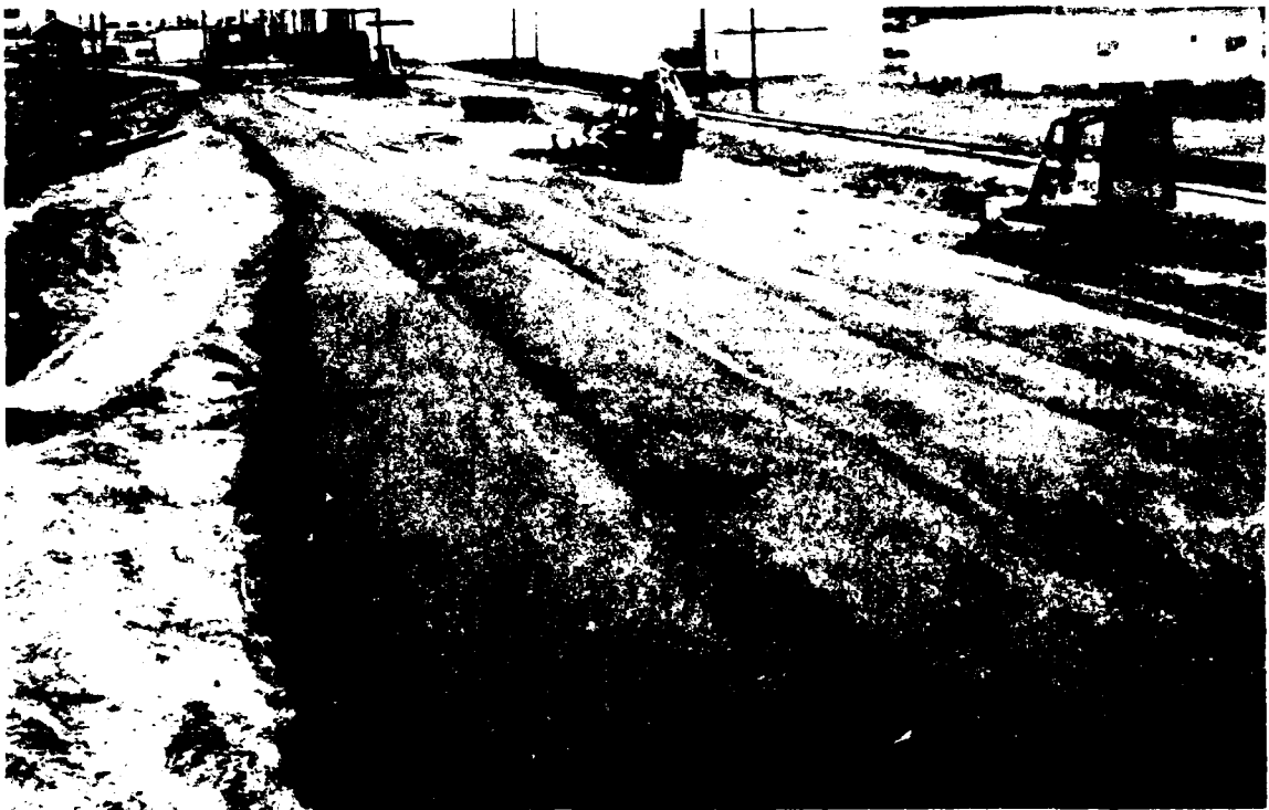
Figure 37. Overall view after asphalt laydown
