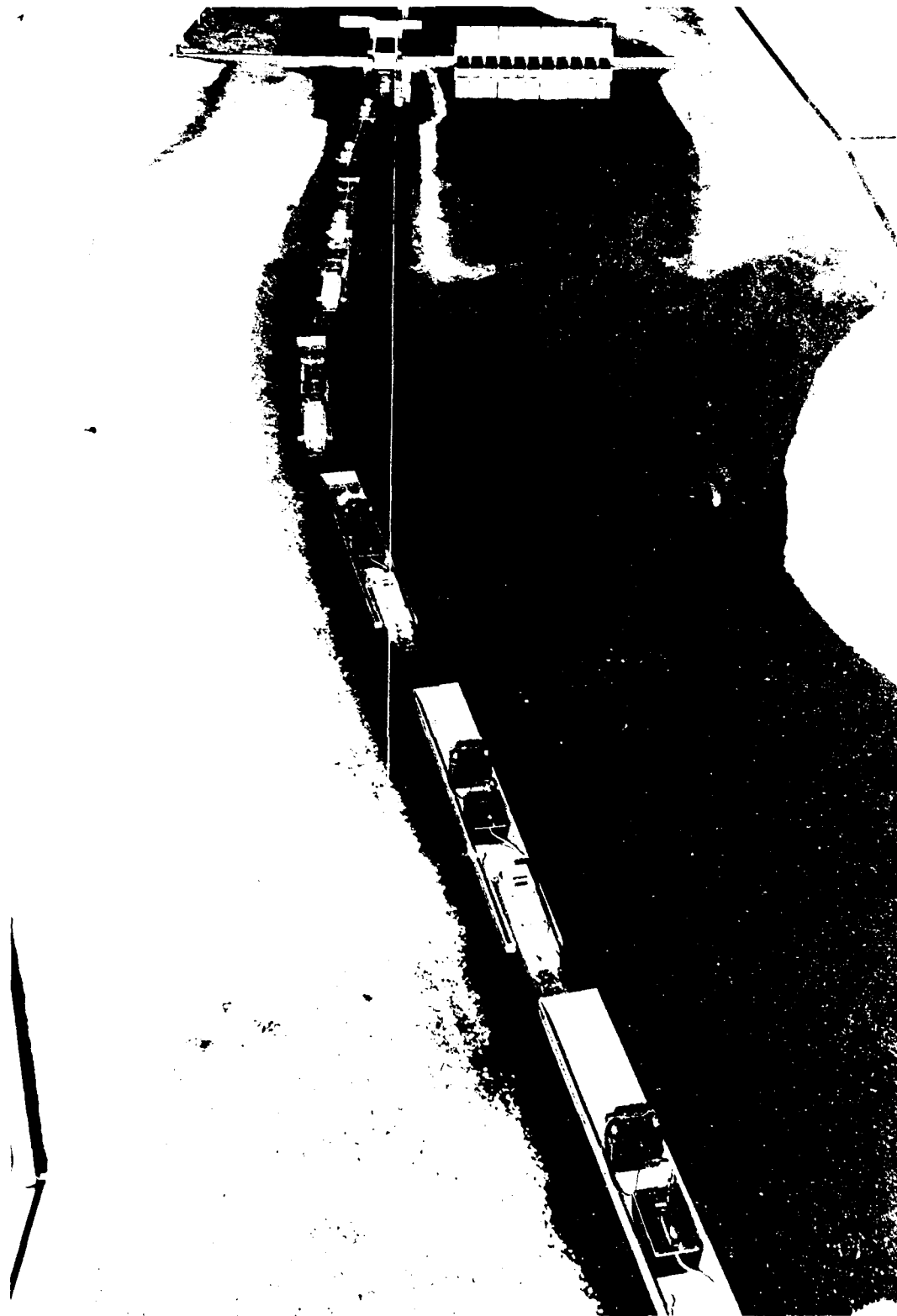
Phot. 4. Plan B-34, downbound tow approaching the canal and lock from upstream; discharge 26,000 cfs, tailwater at 47.2 (normal)
