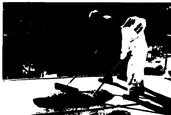
Figure 25. Application of polyester-resin primer
