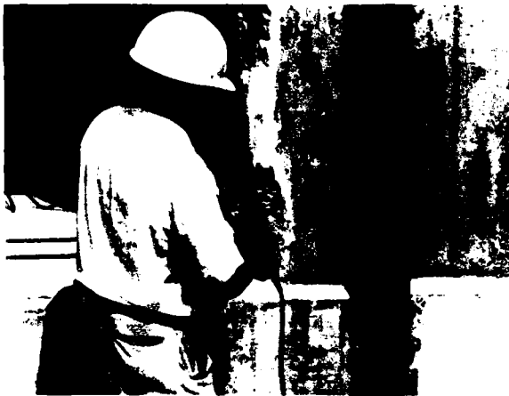
Figure 16. Preparation for vertical spall repair on columns
