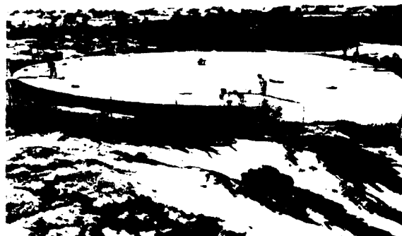
Figure 28. Finished coating on sand trap water storage tank
