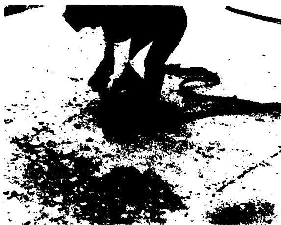
Figure 20. Removal of unsound concrete, Fort Ord
