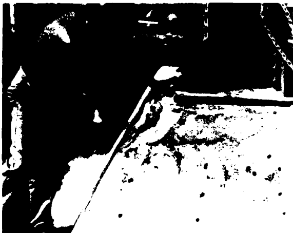
Figure 11. Repair of spalls on concrete footings with latex-modified mortar
