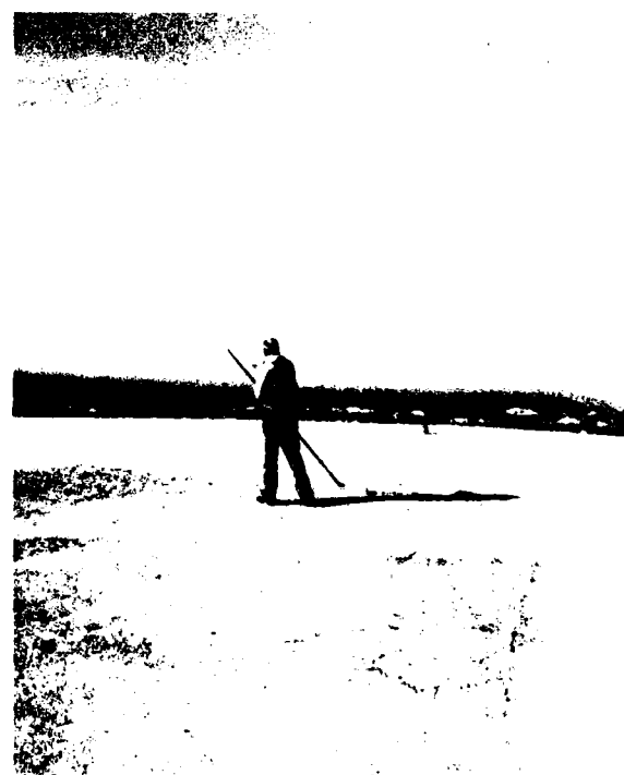
Figure 32. Finishing of slurry coat, reservoir D
