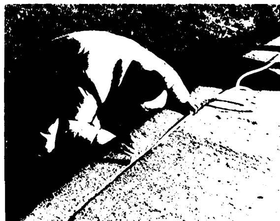
Figure 29. Installation of backing rod in joint
