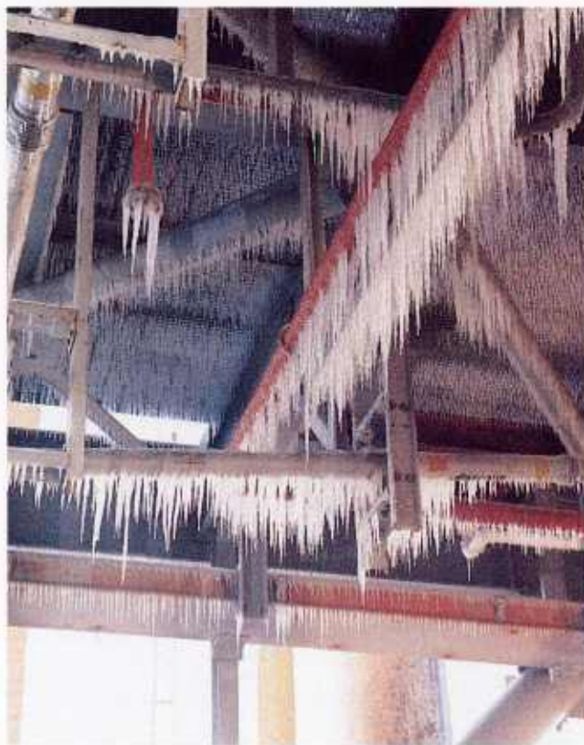
Above, foot long icicles on a lower level of the Fixed Service Structure frame the attachment point where the Orbiter is attached to the external tank (arrow). Icing was even more extensive at upper levels of the service structure (upper right and below). At right below is a ground communications box (not used during launch) rendered inoperable by heavy ice.
