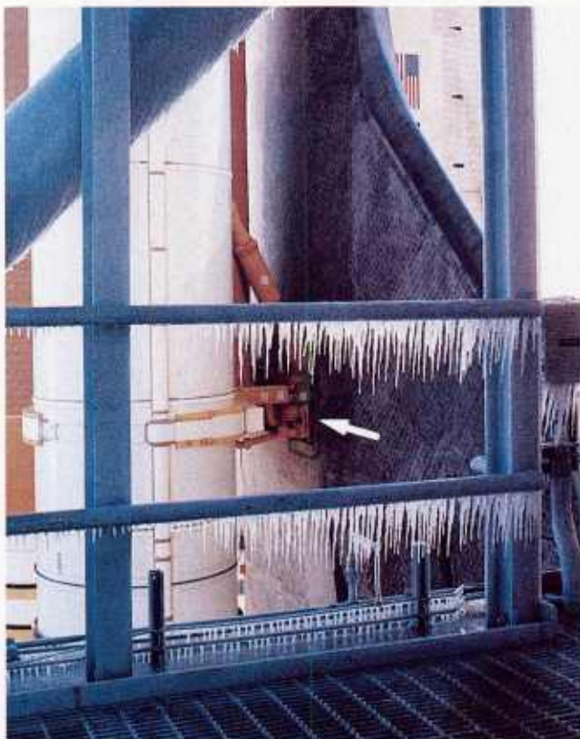
Above, foot long icicles on a lower level of the Fixed Service Structure frame the attachment point where the Orbiter is attached to the external tank (arrow). Icing was even more extensive at upper levels of the service structure (upper right and below). At right below is a ground communications box (not used during launch) rendered inoperable by heavy ice.
