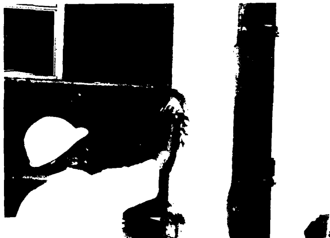
Figure 5. Spalled area, primer being applied
