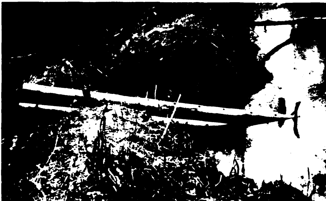
Figure 3. View of an uncovered, perforated plastic 3-pipe drain installed in a beaver dam break
