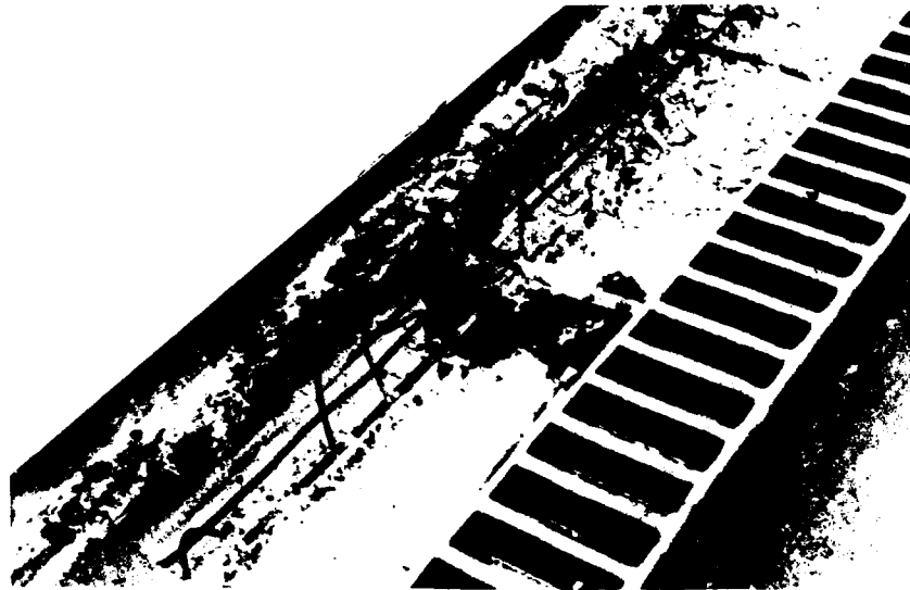
Figure 10. Gate recess area after removal of concrete between waterside rail and rack. Note the rods which serve as lateral stiffeners of the rail-support girder
