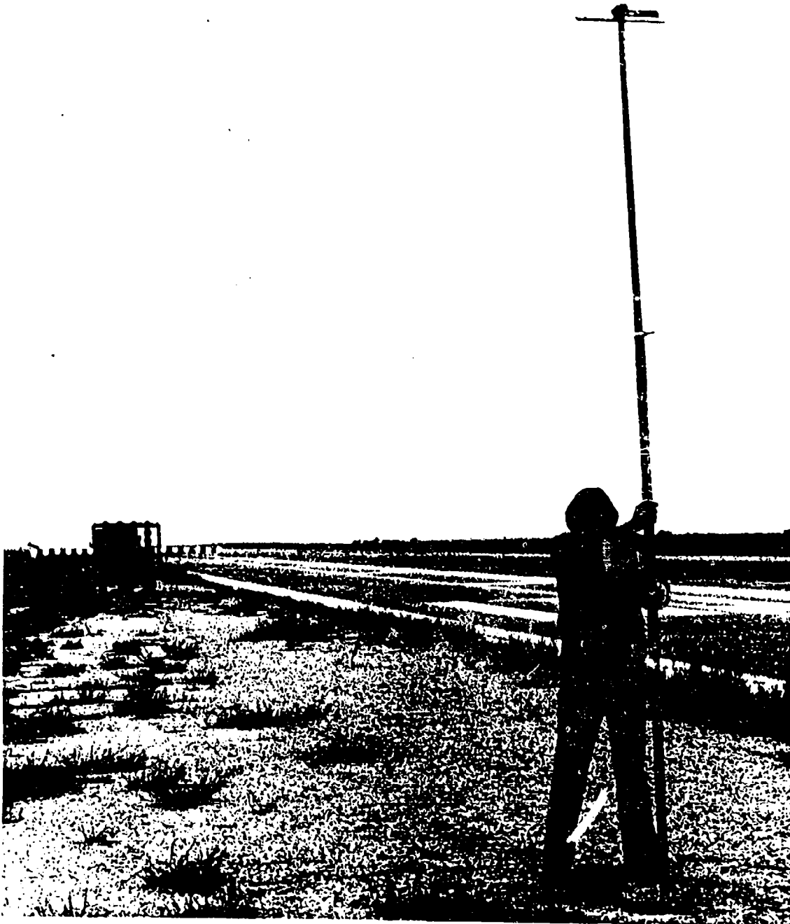
Figure C-5. FLOLS Calibration Procedure Used by Landing Signal Officers to Set the FLOLS Glideslope
