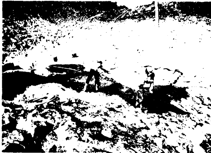
Photo 54. Placing and vibrating dental concrete in Stage I core trench. 10 February 1984
