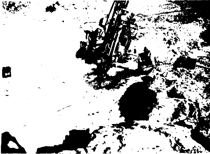
Photo 73. Drilling first zone of primary grout hole 30+00P using air track percussion drill. Air-water mixture used as circulating medium. 10 January 1984
