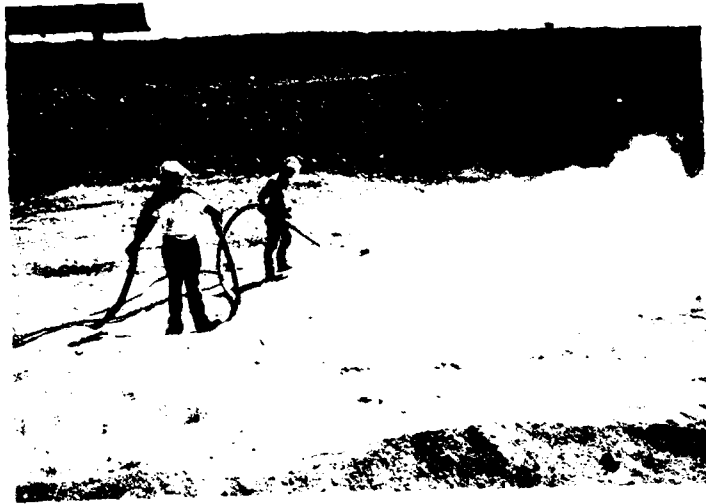
Photo 65. Air cleaning core trench surface at station 20+80 using high pressure bull hose. 16 March 1984
