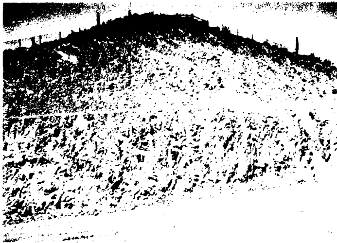
Photo 95. Typical example of strongly jointed andesite flow exposed in north wall of spillway excavation, vicinity station 17+00. Note variable joint patterns and darker colored "zone of weathering" near surface of flow. 20 March 1985
