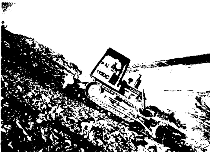
Photo 42. Case 1150C dozer ripping right abutment with double shank ripper teeth; note double parted winch cable. 6 December 1983
