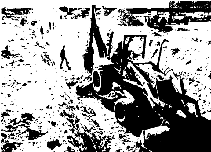
Photo 84. Foundation preparation of outlet conduit excavation using backhoe and hand labor. 18 January 1984
