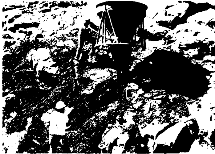
Photo 59. Placing dental concrete on right abutment slope using concrete bucket. 2 October 1984
