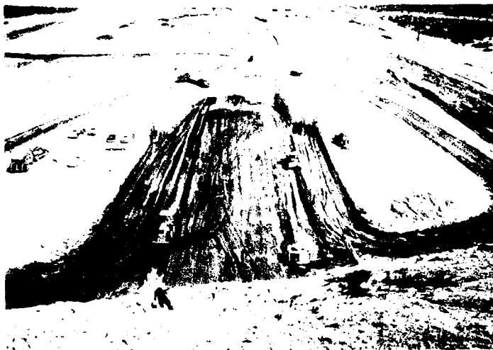
Photo 17. Stage I dam embankment fill placement. Note breach in Stage I diversion levee to allow equipment access. 28 February 1984
