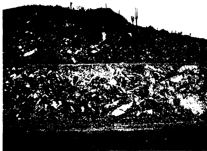
Photo 107. South wall of completed spillway excavation, vicinity station 16+00. Note variable joint orientations and spacings, including prominent dip-slope joint planes. 18 April 1985
