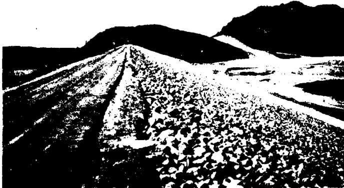
Photo 2. View of dam embankment crest and upstream face looking toward right abutment. 20 March 1985
