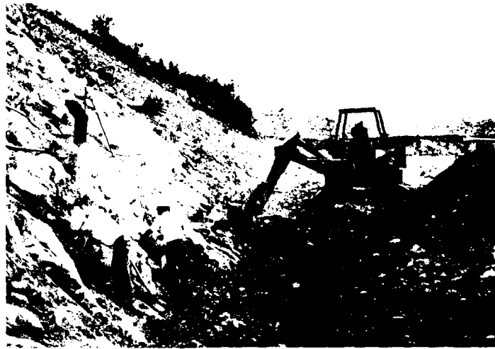
Photo 57. Beginning Stage III right abutment surface preparation. Laborers permitted to work only short reaches without safety lines. Note backhoe removing Stage I protective cover down to elevation 1380 near base of slope. 29 September 1984
