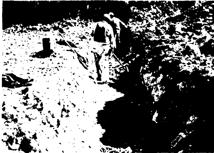
Photo 105. Laborers cleaning loose rock from invert section of spillway sill. Variable bedrock structure resulted in wider and slightly deeper excavation than originally designed. 29 November 1984
