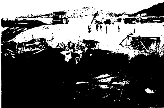
Photo 114. Front end loader compacting core material against bedrock slope in Stage II core trench, vicinity station 16+50. Note dozer using blade to spread core material over foundation surface. 2 April 1984
