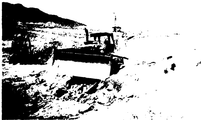
Photo 68. D9H dozer using slopeboard to flatten bedrock slope near station 16+50 to 1:1 and remove soft weathered bedrock from foundation surface. 12 March 1984
