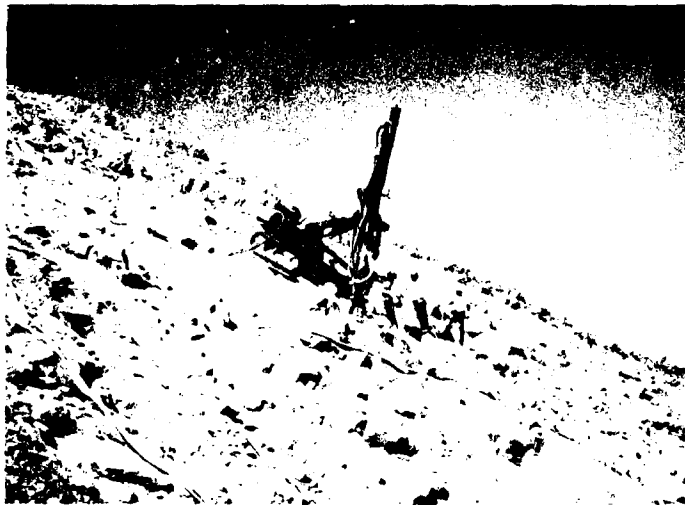
Photo 74. Air track drilling first zone of secondary grout hole 32+34S on right abutment slope. Drill pulled up slope using winch cable system. 6 March 1984
