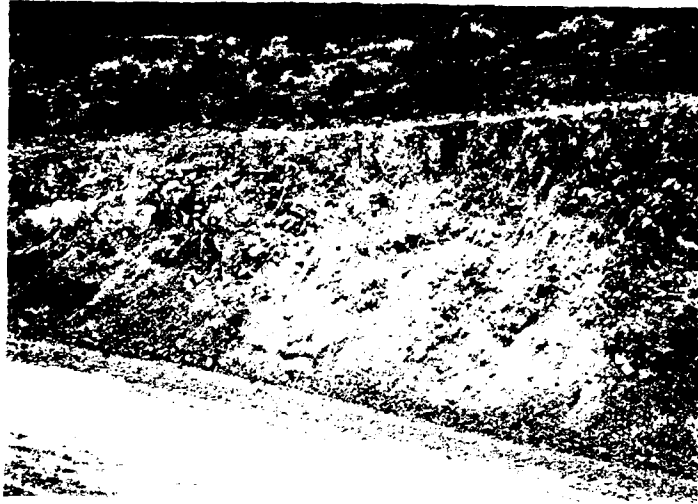
Photo 117. Slope failure in intensely fractured platy andesite, north wall of spillway excavation, vicinity station 14+00. 18 April 1985
