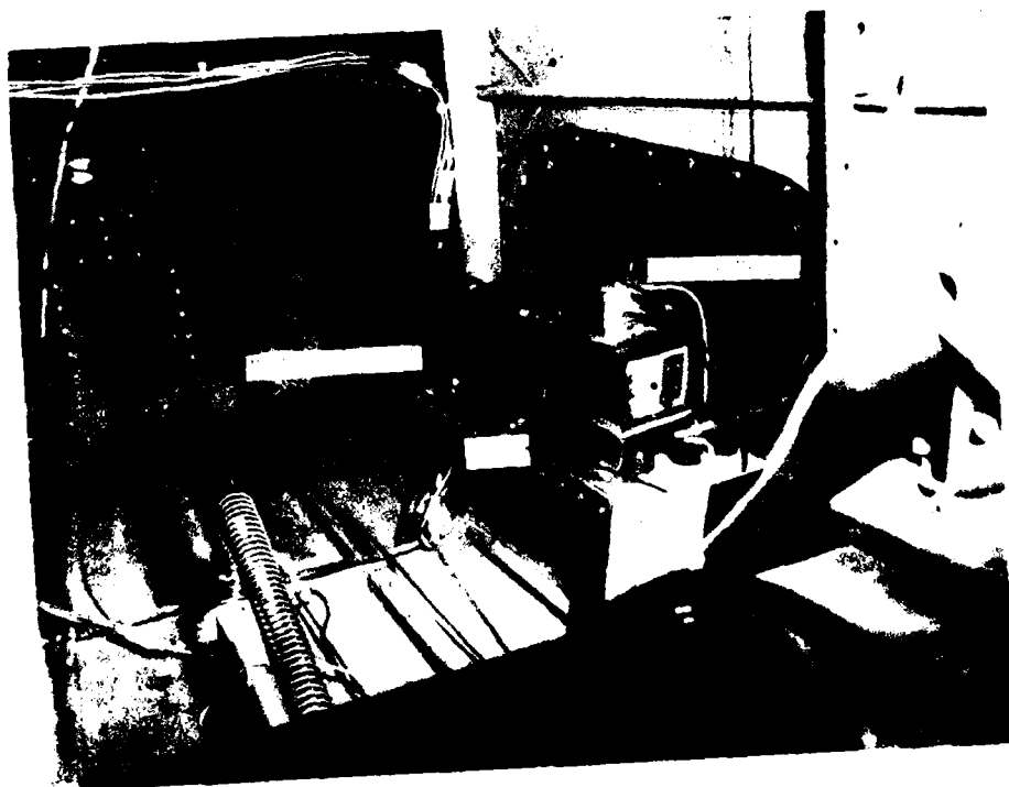
Figure 16. Typical NASA-Langley Research Center emergency locator transmitter (ELT) installation.
