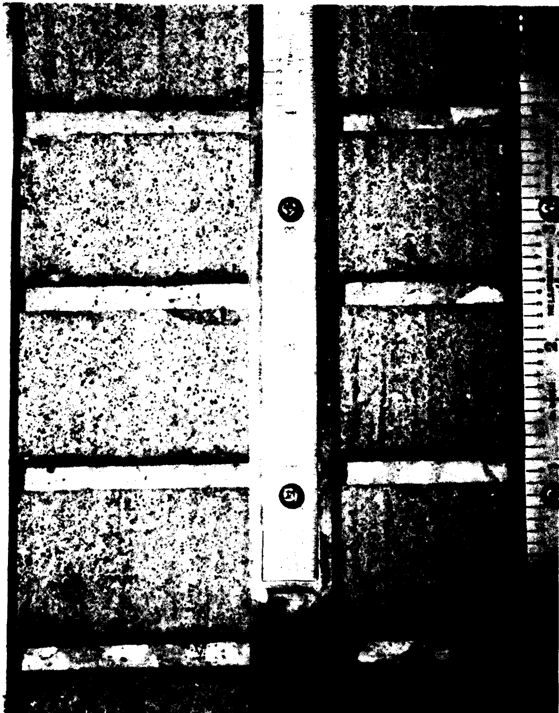
FIGURE B-1. RUNWAY Q, A GROOVED PORTLAND CEMENT CONCRETE (RUNWAYS C, E, G, AND P SIMILAR)
