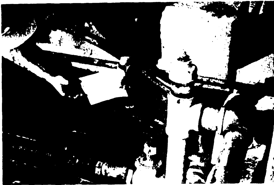
CORRODED CONDITION OF DECK, STRINGERS ON PIER D-1 FINGER PIERS. NOTE KNIFE BLADE THROUGH BEAM WEB.
