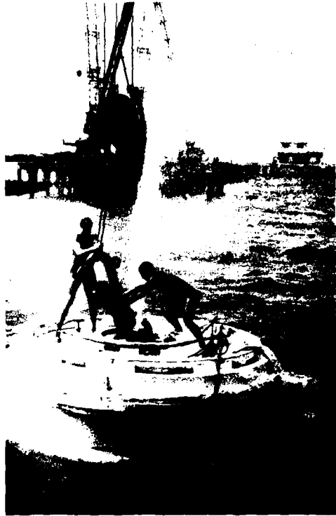
No. 14 Buoy - raised - all chains connected underwater - mooring shackle attached
