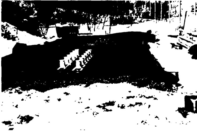
Figure 1. Forms for slabs 1 and 2. Push-out molds are in place prior to placing of concrete.
