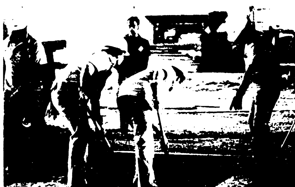
Figure 7. Working and screeding the patch material
