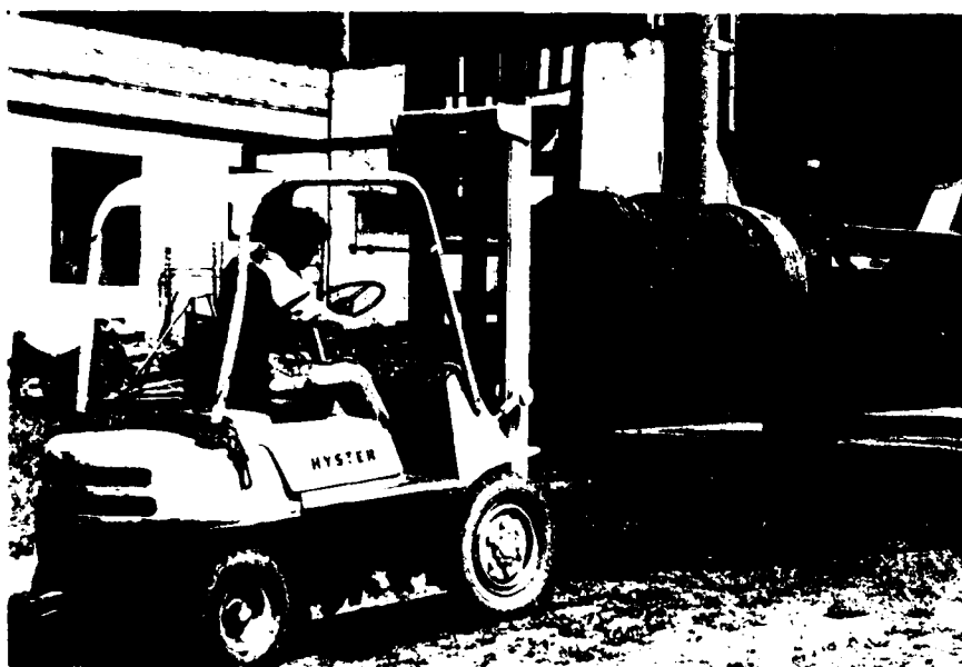
Figure 6. Threading truck tires onto steel pipe
