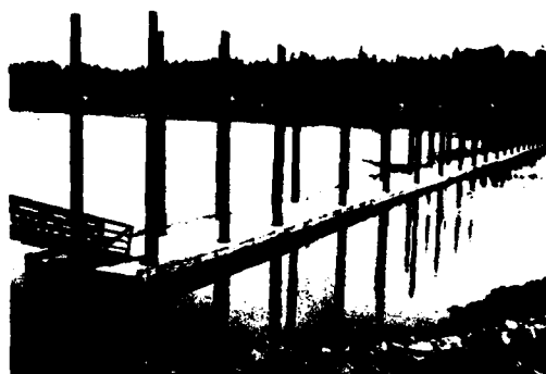
PHOTO 25. THE 16-FT-WIDE BY 600-FT-LONG EAST BAY BREAK- WATER MOORED WITH PILINGS
