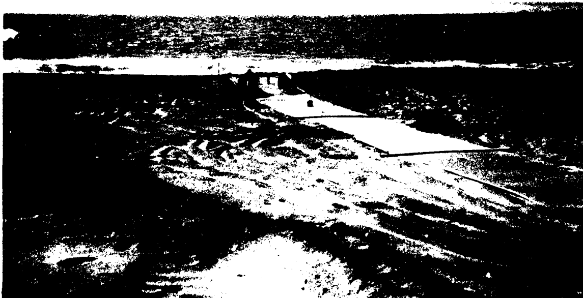
Figure 4-10. Beach matting for split-pipe application and haulout.
