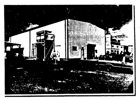
Figure  $4_{-3}$ . Building 223 Hill AFB PRAM plastic media paint stripping facility. On the left is one of two air ventilation dust collectors. The rollup door provides access to the mechanical equipment room. The main access door is located at the opposite end of the facility.
