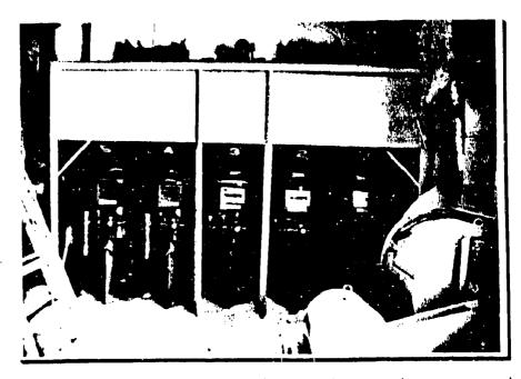
Figure 4-4 - Equipment Room. Plastic media storage hoppers mounted above Paulli and Griffin blasting machines.
