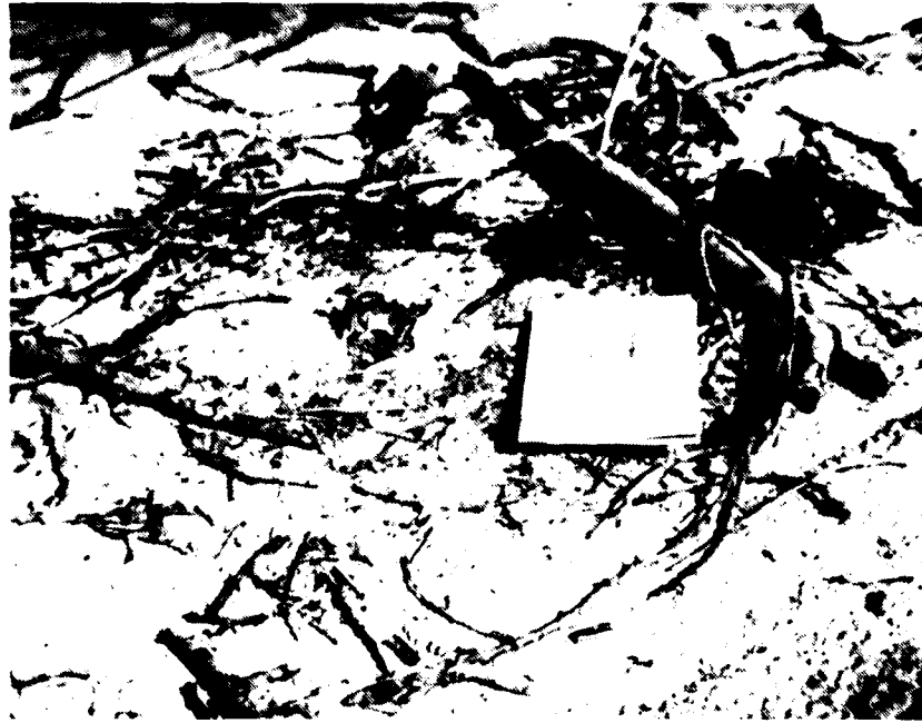
Figure 13. System 1 - Acrylic elastomer without granules. Severe accumulation of dead tree limbs and leaves; plants growing in punctures. Naval Station, Roosevelt Roads, P.R.
