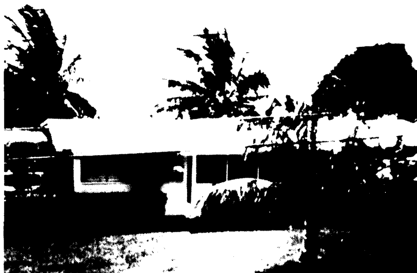
Figure 1. Typical experimental house with low slope concrete roof deck. Note tropical foliage, which is often dense, and roof mounted TV antenna. Naval Station, Roosevelt Roads, P.R.
