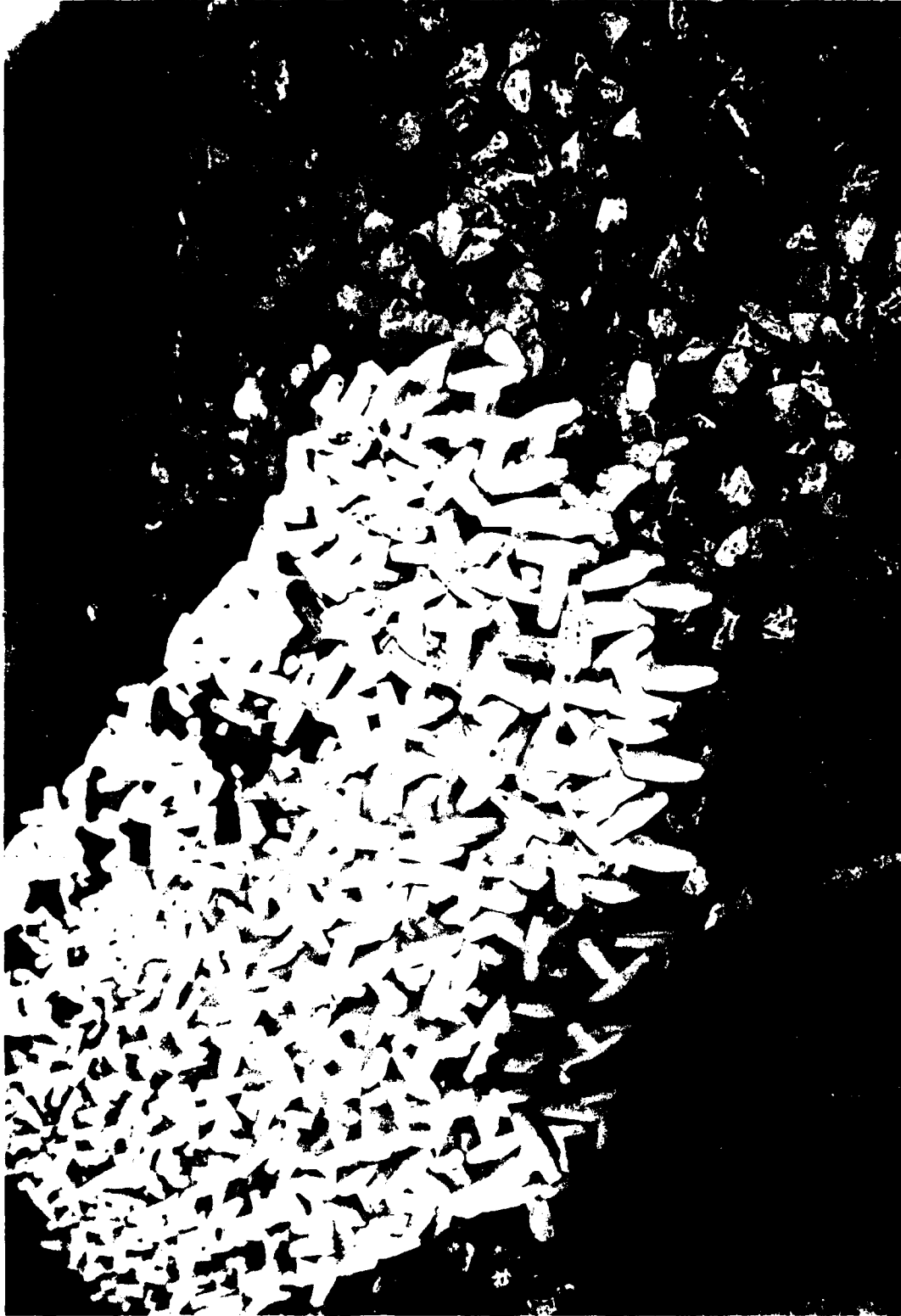
Photo 29. Special toe placement used for seaward transition of Plan 2B
