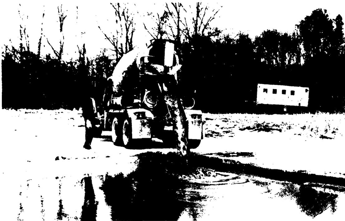
Photo 1. Placement of grout in crater
