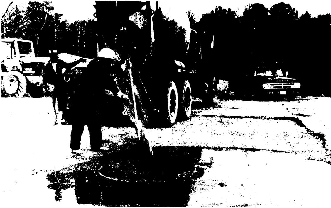
Photo 13. Placing grout cap on limestone
