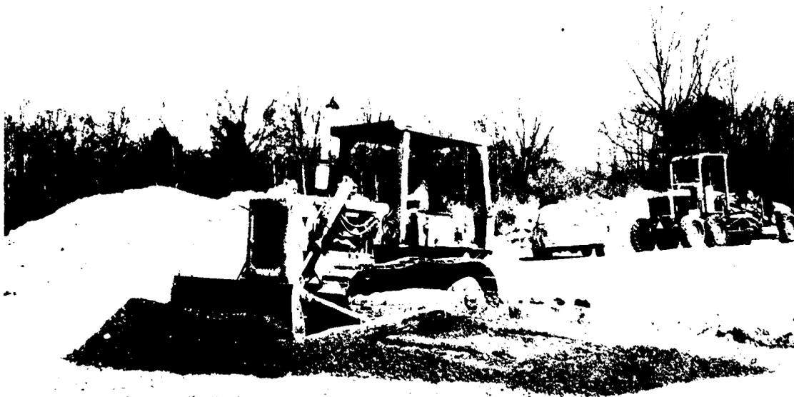
Photo 6. Spreading stabilized material in crater 3
