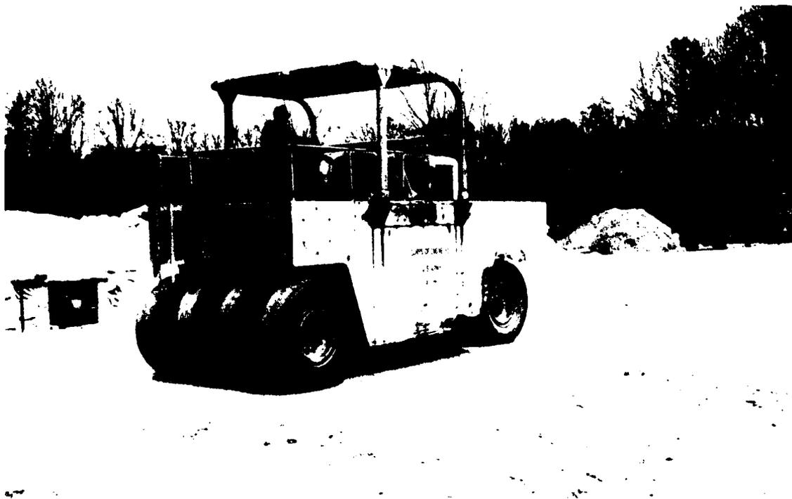
Photo 10. Rolling the sand placed over the AC-20
