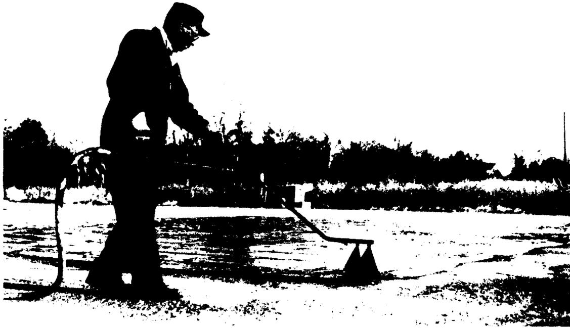
Photo 9. Bituminous seal being applied to crater 3
