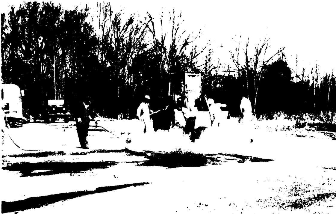
Photo 17. Spraying AC-20 and spreading limestone
