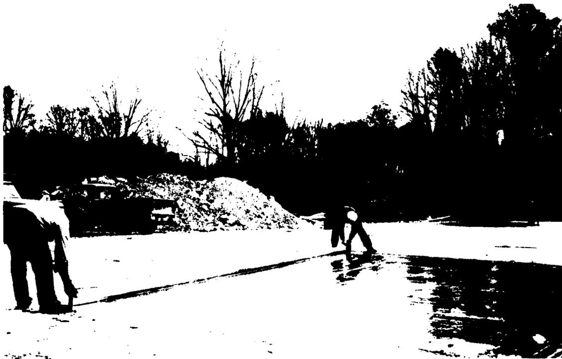
Photo 14. Moving and leveling grout in crater 4
