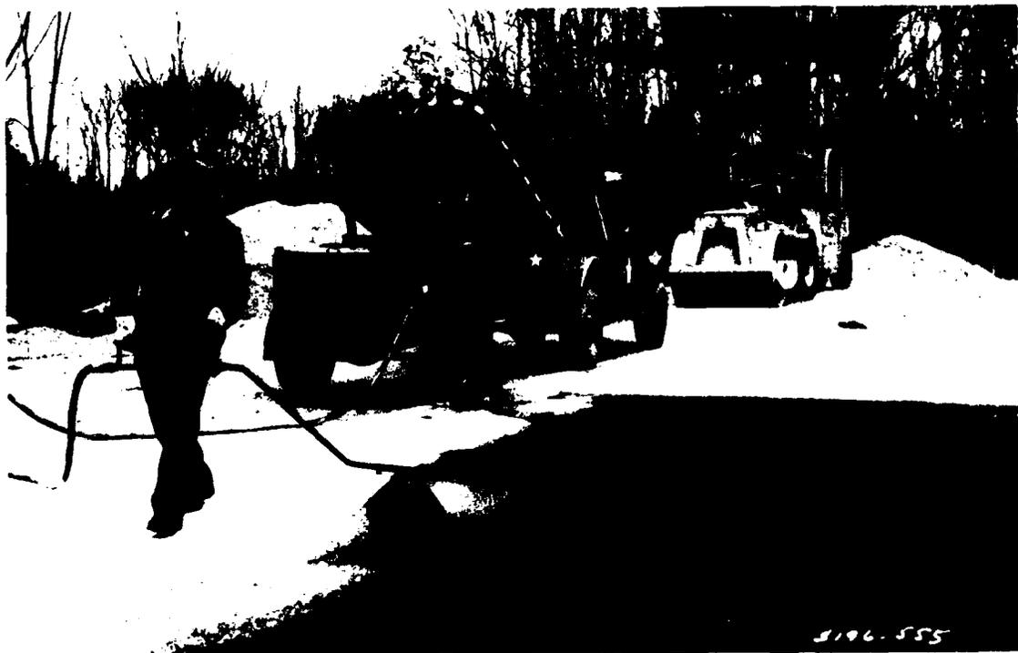
Photo 16. Priming the surface of crater 5
