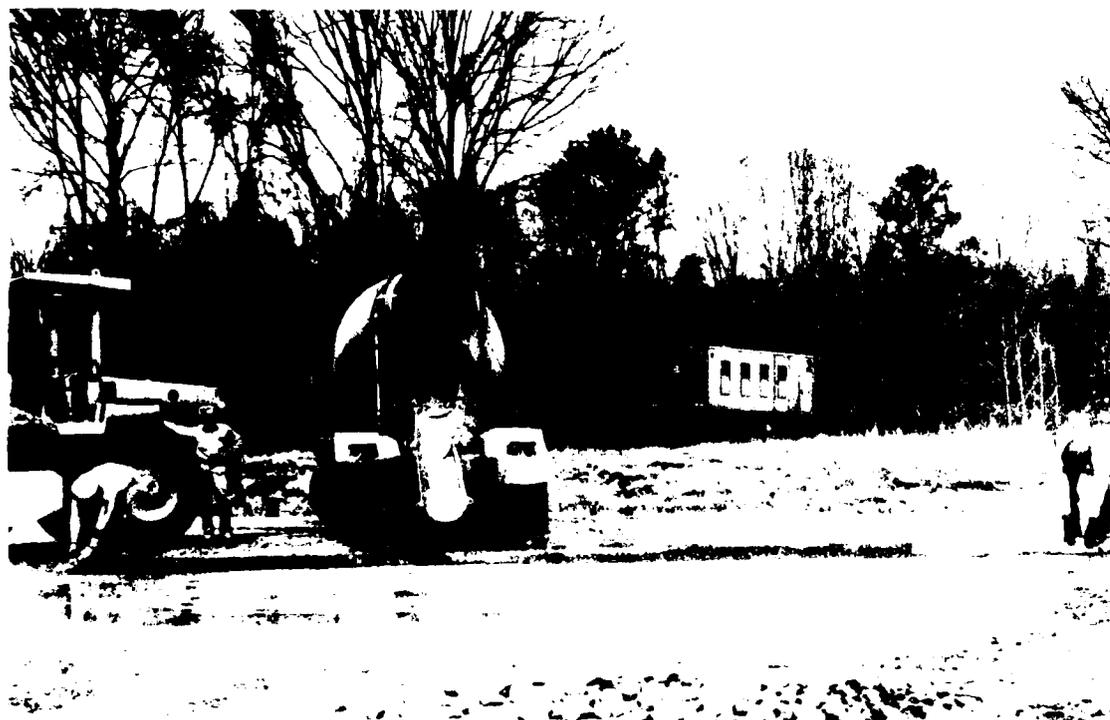
Photo 4. Spreading and leveling the grout
