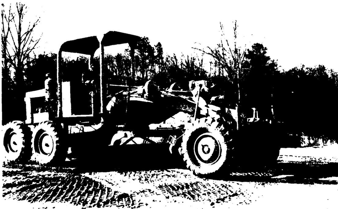
Photo 8. Leveling the surface of crater 3
