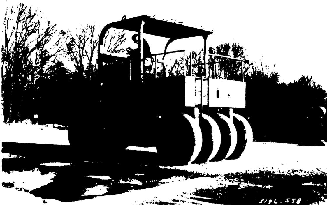
Photo 18. Embedding the limestone into the AC-20
