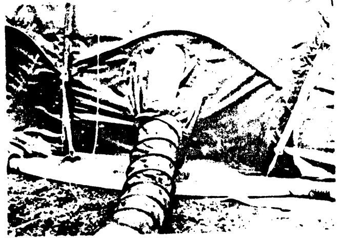
Figure 53. Environmental control duct entering shelter (outside)
