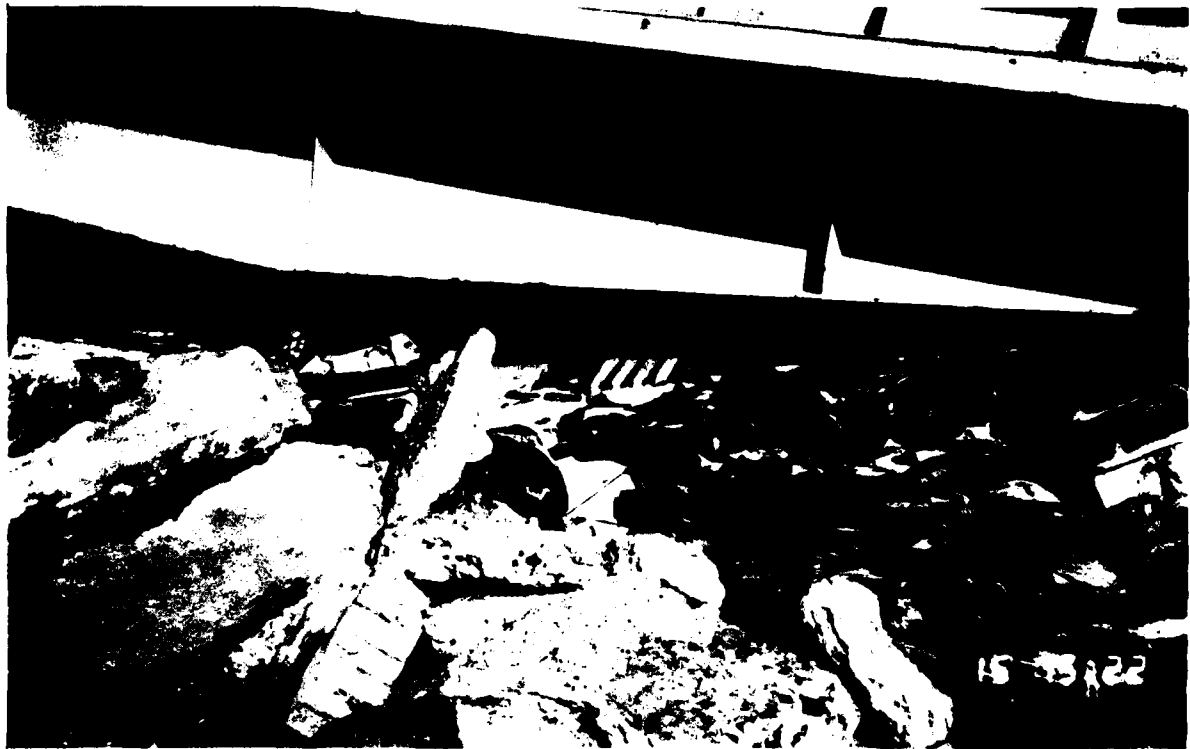
Figure 5-6 - Rubble Protection for DeLong Ramp Abutment
