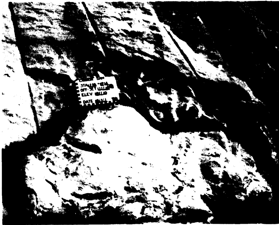
Station 18+74, Offset 115 feet upstream, Elevation 610 feet. Final foundation of left abutment. 31 May 1983
