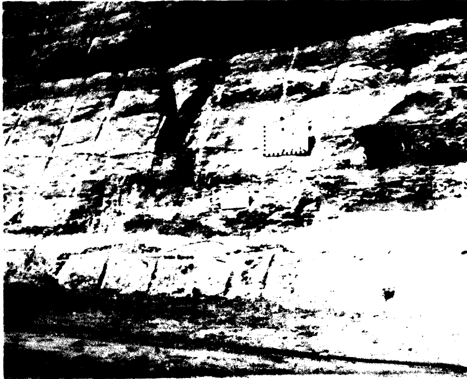
Station 18+12, Offset 140 feet downstream, Elevation 575 feet. Final foundation of left abutment in sand drain zone. 9 Sept. 1982.
