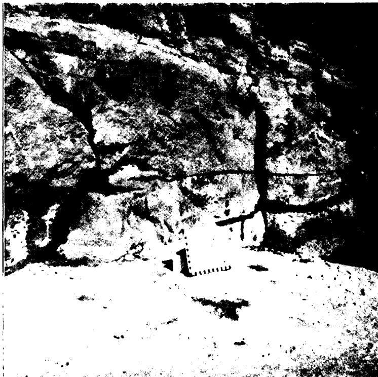
Station 17+80, Offset 392 feet downstream. Elevation 563 feet. Final foundation left abutment. 6 Oct. 1980.
