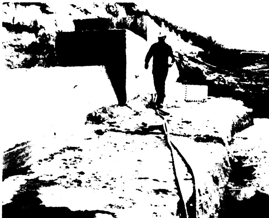
Station 17+90, Offset 400 feet upstream, Elevation 570 feet. Looking downstream at final foundation of left abutment. 15 Sept. 1981.
