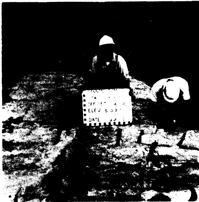
Station 15+70, Offset 40 feet downstream, Elevation 503.5 feet. Final shale foundation in Diversion Channel. 25 Sept. 79.
