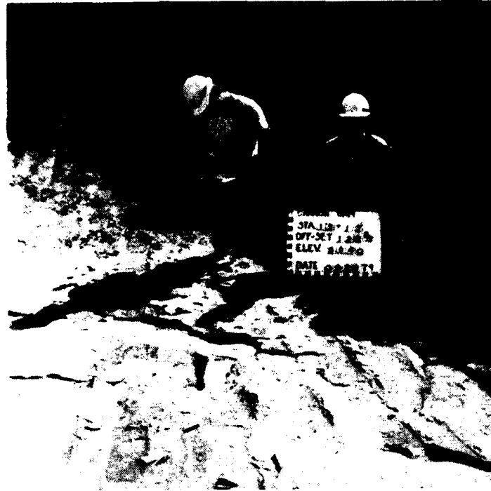
Station 15+17, Offset 128 feet downstream, Elevation 504 feet. Final shale foundation in Diversion Channel. 28 Sept. 79.
