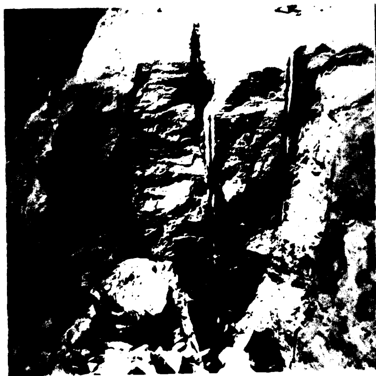
Left abutment cutoff wall excavation. production shot from elevation 590-600 feet. Note degree of fracturing. 12 April 1978.
