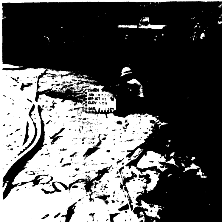
Station 16+70, Offset 45 feet upstream, Elevation 509 feet. Final shale foundation in Diversion Channel. 14 September 1979
