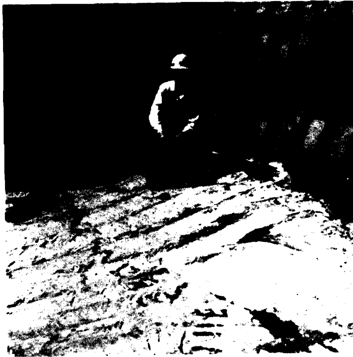
Station 15+74, Offset 95 feet upstream, Elevation 504.3 feet. Final shale foundation in Diversion Channel. 24 Sept. 1979.
