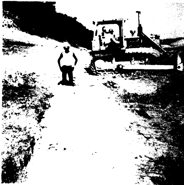
Station 16+56, Offset 160 feet downstream, Elevation 509.1 feet. Final shale foundation in Diversion Channel. 17 Sept. 79.
