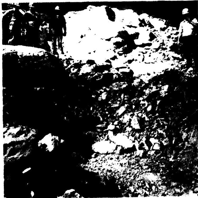
Left abutment cutoff wall excavation, production shot from elevation 590-600 feet. View to the north. 11 April 1978.
