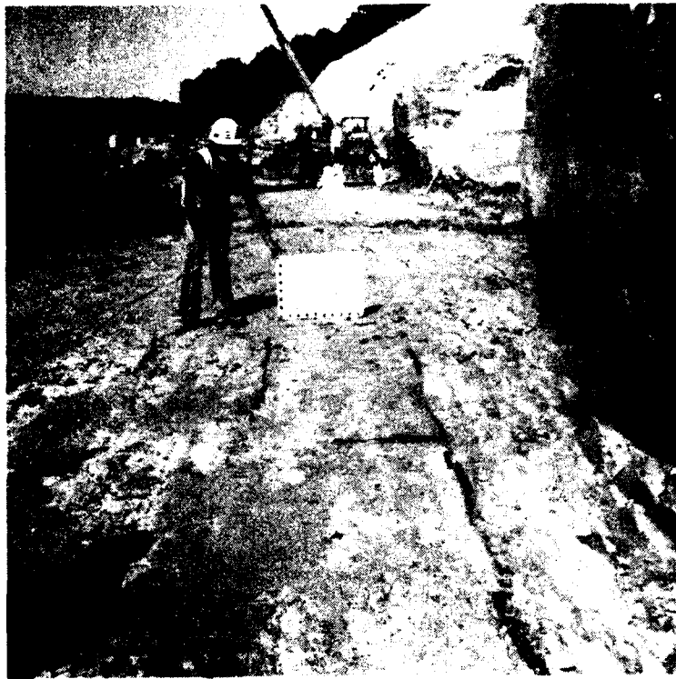
Station 17+71, Offset 344 feet downstream, Elevation 549 feet. 27 July 78. Left abutment shale preparation for fillet placement, final foundation. Joint set: Strike N76E, Dip vertical, average spacing 0.2 feet to 0.5 feet.
