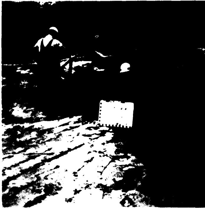
Station 16+29, Offset 76 feet upstream. Elevation 504.3 feet. Final shale foundation in Diversion Channel. Note joint face in background. 20 Sept. 79.
