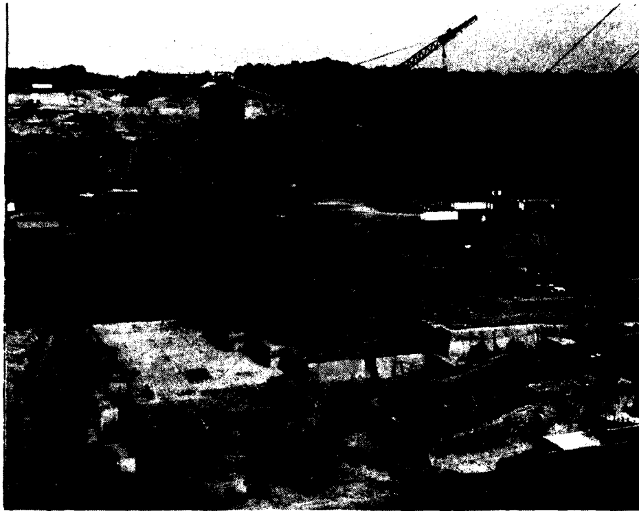
Main dam excavation, left abutment in background. October 1974.
