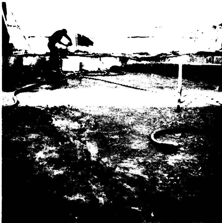
Station 6+20, Offset 15 feet upstream, Elevation 464 feet. Final foundation, Powerhouse. 16 May 1975.
