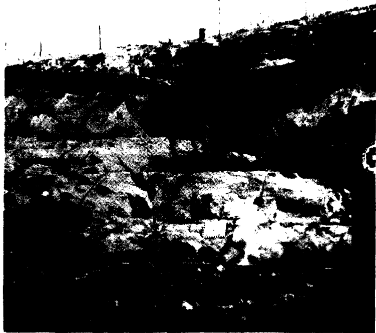
Station 2+10, Offset 201 feet downstream, Elevation 602 feet. Right abutment. 28 November 1973.
