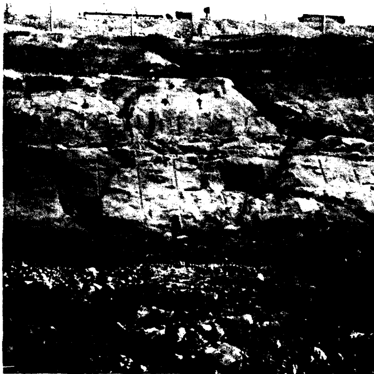
Station 2+10, Offset 125 feet downstream, Elevation 602 feet. Right abutment. 28 November 1973.
