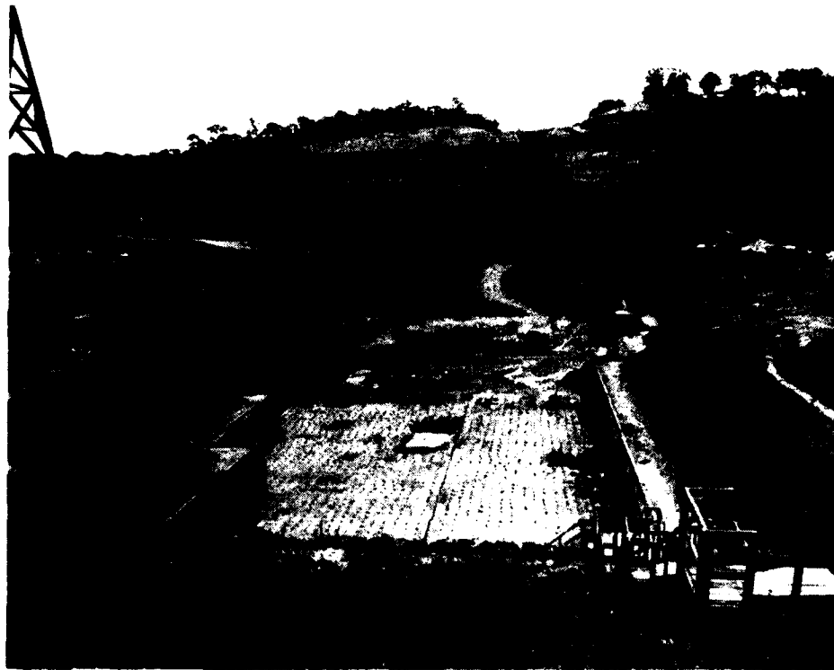
Excavation of foundation for Main Dam and Right Abutment. Oct. 1974.
