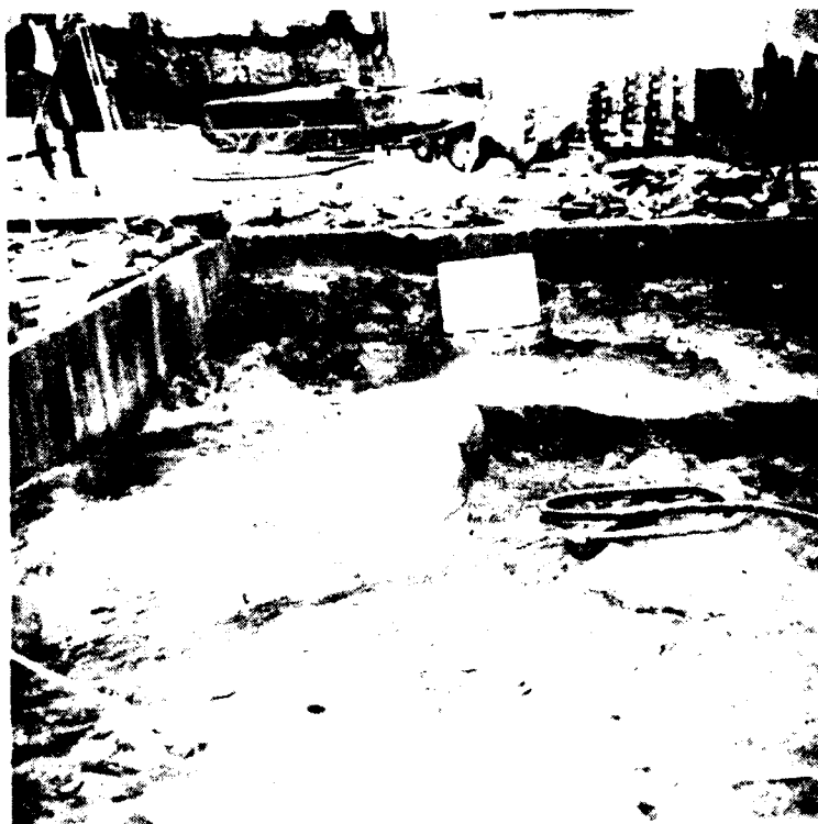
Station 7+60, Offset 10 feet upstream, Elevation 464 feet. Final foundation, Powerhouse. 9 May 1975.
