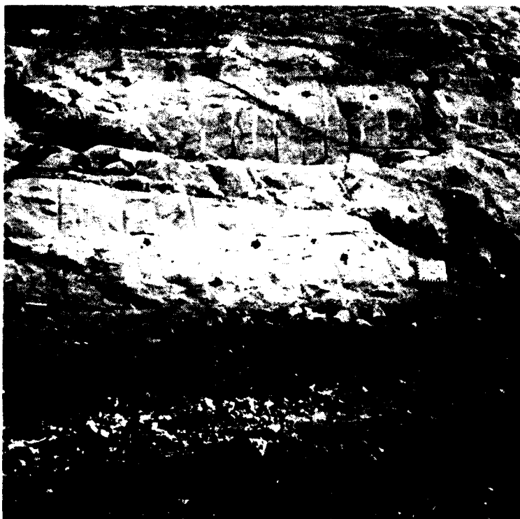
Station 2+10, Offset 101 feet downstream, Elevation 602 feet. Right abutment. 28 November 1973.
