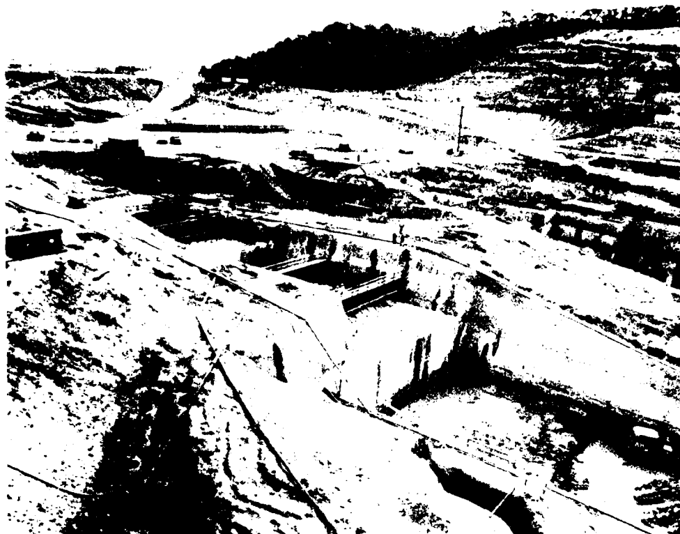
Photograph E. Picture showing dewatering operations. Note header lines used to carry water to main sump. Pooled water on floor of tailrace wall foundation was removed using small portable trash pumps.
