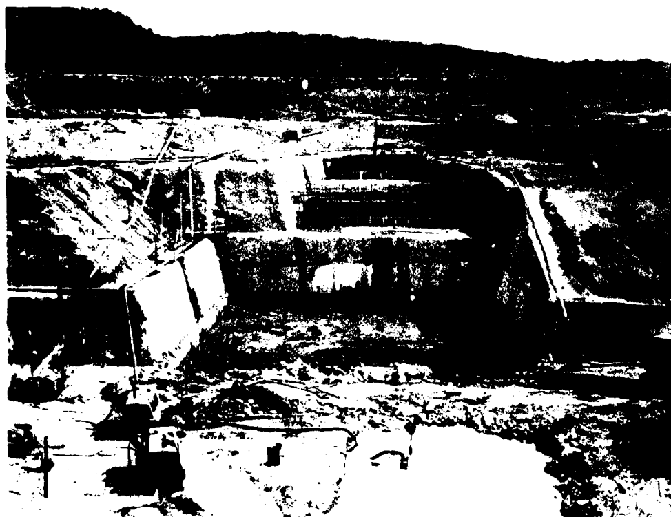
Photograph F. Picture showing dewatering operations in concrete structure. Note large dewatering pump in foreground. Second stage cofferdam in background.
