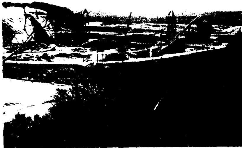
Photograph C. Overall view of dewatering operations in concrete structure. Note interceptor ditch which lies above 4851 berm on upstream and north sides of excavation.
