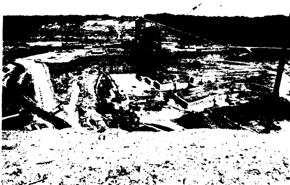
Photograph B. Overall view of concrete structure. Note 4851 berm at base of exposed shale. Pounded water on floor of structure was removed using small portable trash pumps and pumped to main sump.
