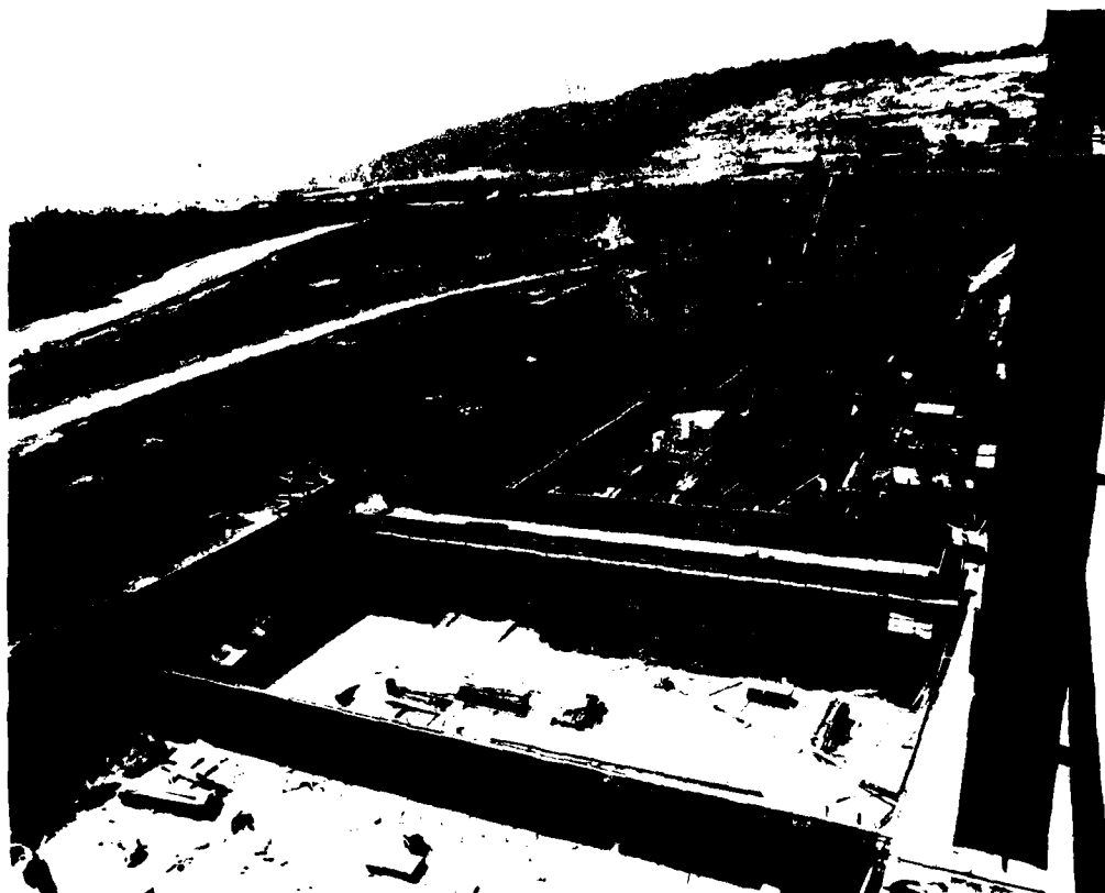
Photograph D. Overall view of dewatering operations in concrete structure. Note header lines used to carry water back to main sump. Lines extend from base of excavation over downstream walls of excavation.
