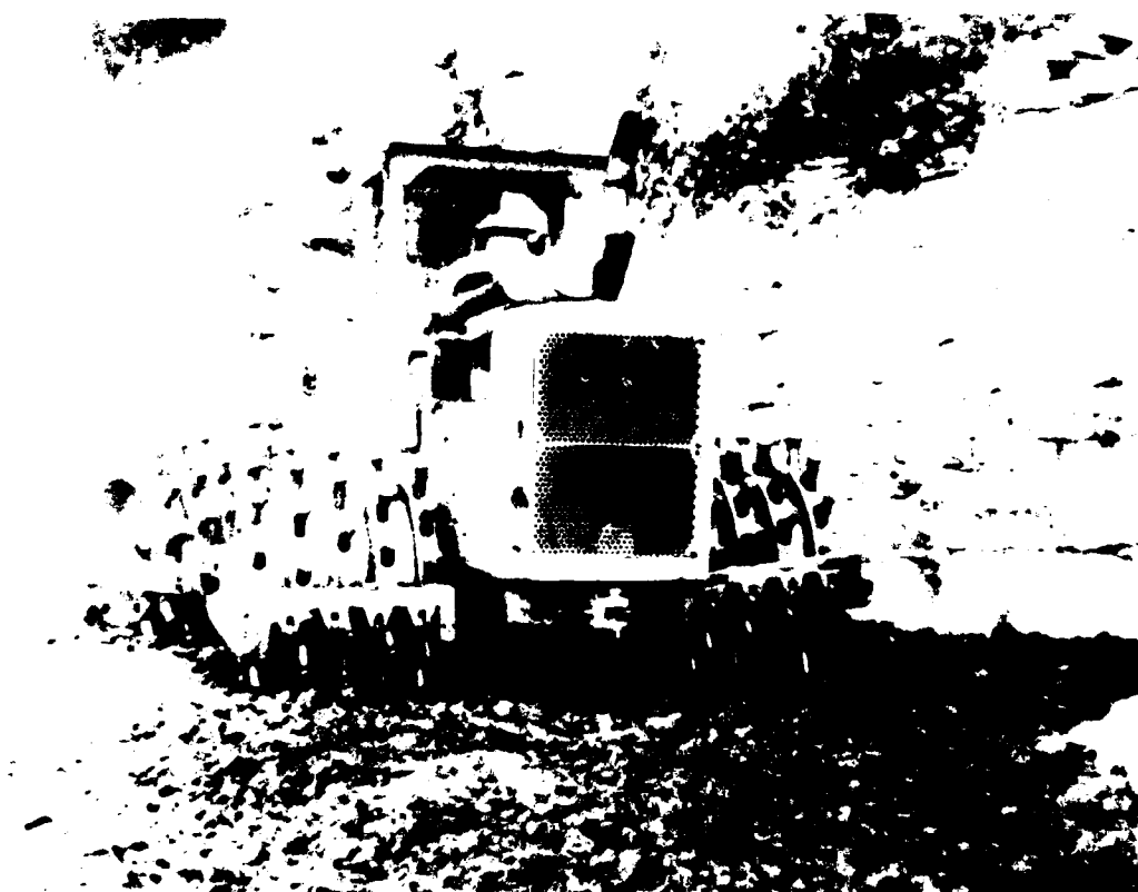
Photograph D showing rolling of fill using sheepfoot roller near rock/empankment contact of water temperature control weir.
