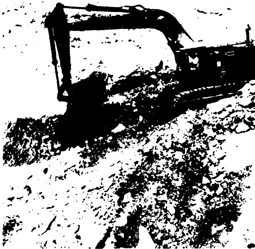
CAT 245 backhoe excavating shot rock from back (north) slope of the cutoff trench.
