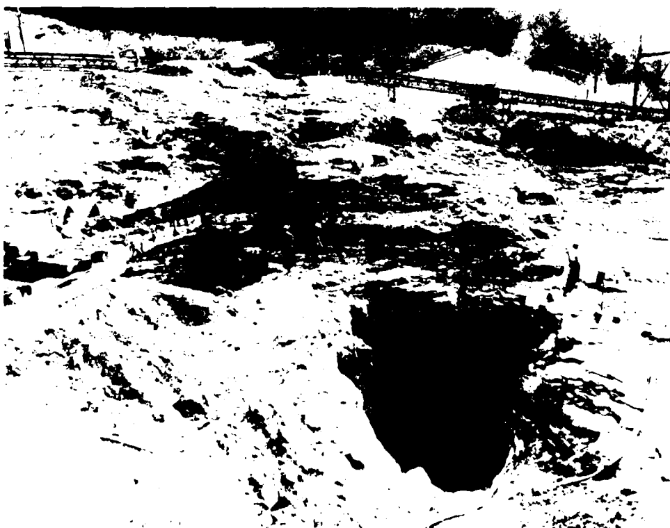
Left Abutment Cutoff Trench, Exposure of Cavities Nos. 1 and 2
