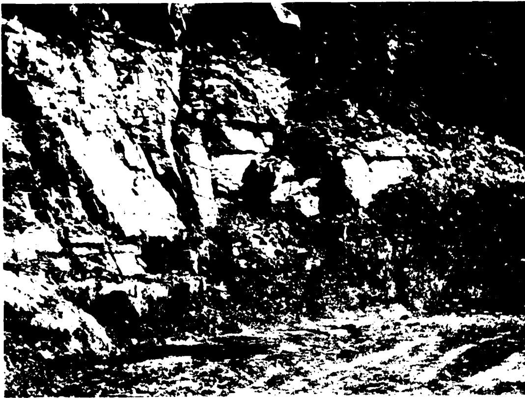
Photograph A depicting condition of rock before treatment is performed on right abutment water temperature control weir embankment/rock contact.
