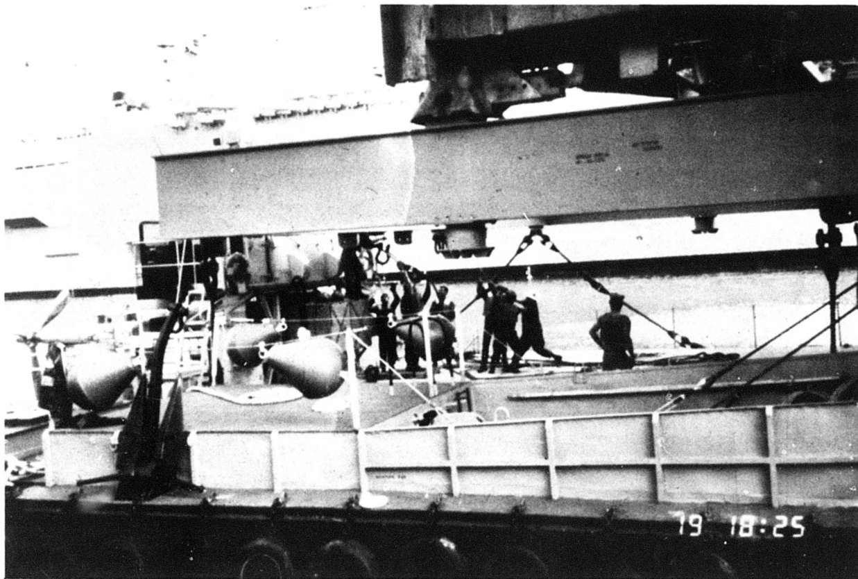
Figure 81 - Attaching LACV-30 Sling to CLF from the Deck of the LACV-30
