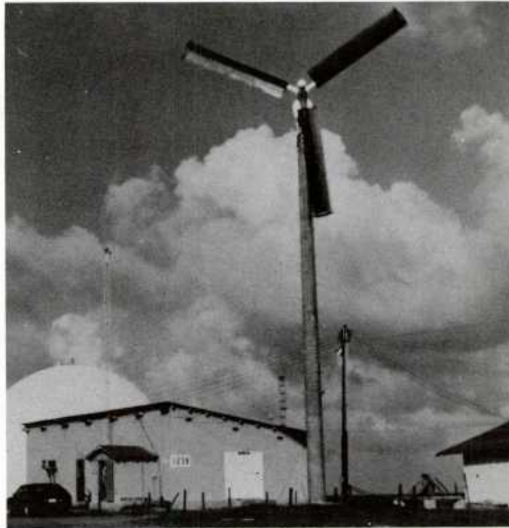
Figure 25. 20-kW WECS installed at MCAS Kaneohe Bay, Hawaii.
