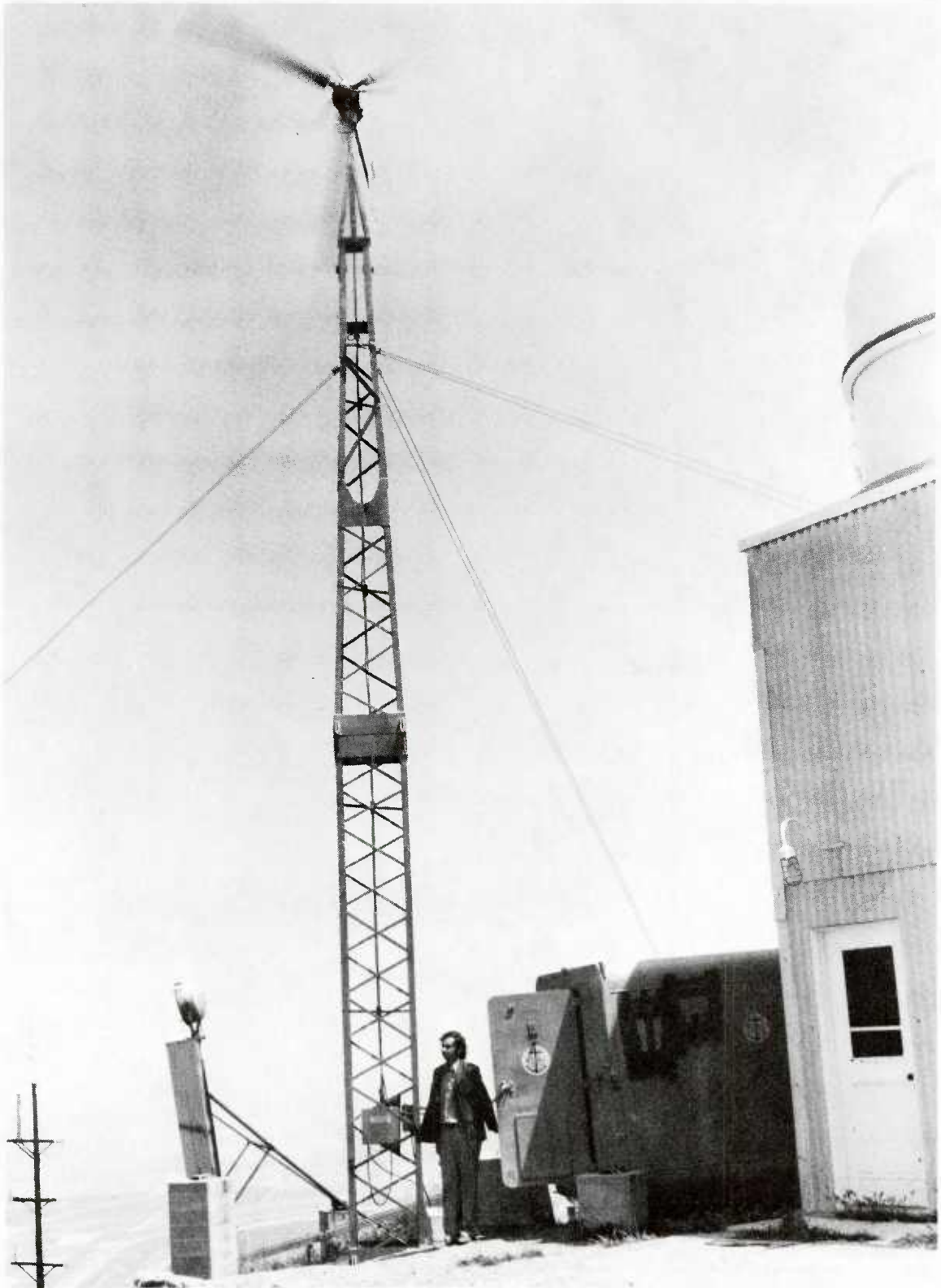
Figure 8. 5-kW WECS installed at San Nicolas Island.
