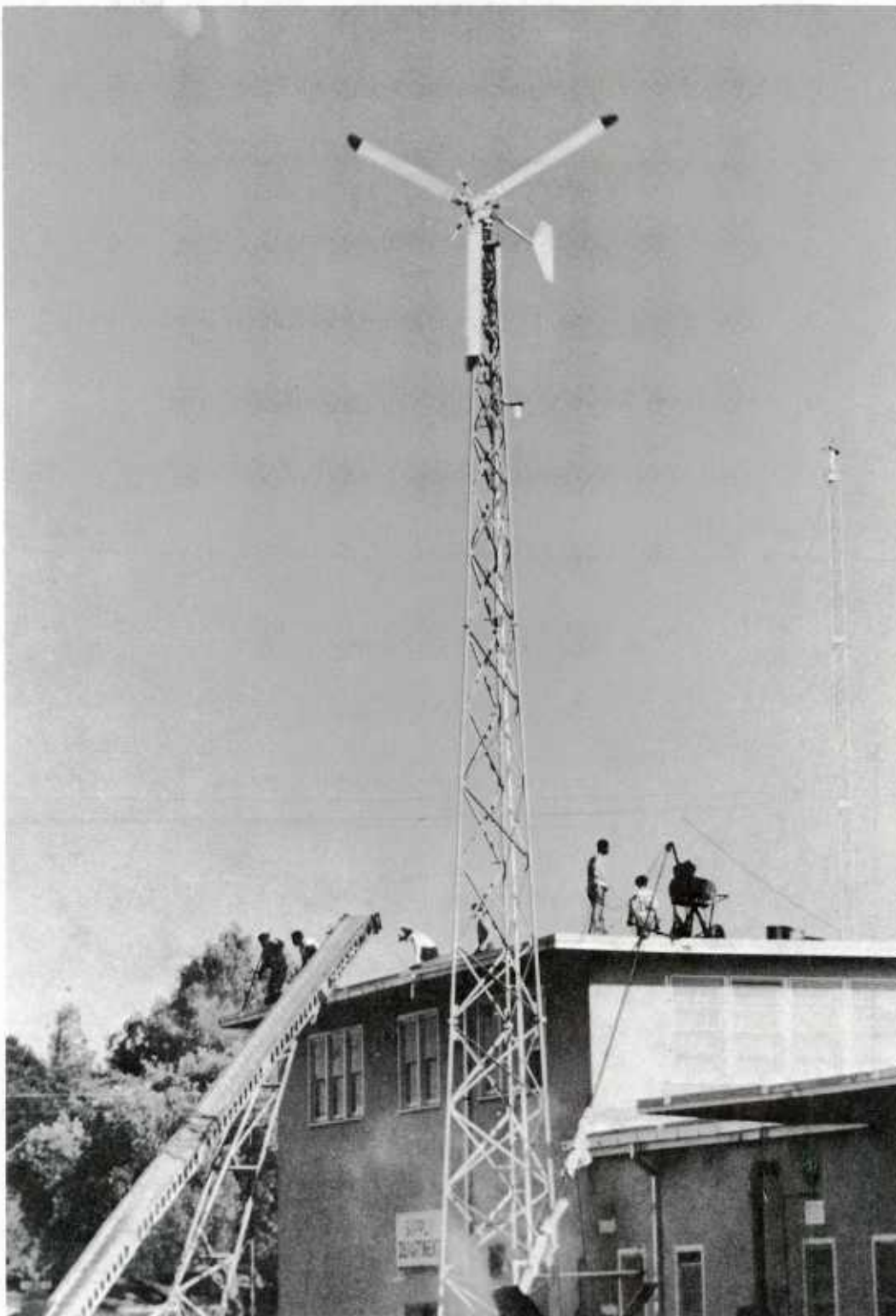
Figure 11. 6-kW WECS installed at Naval Station, Treasure Island.
