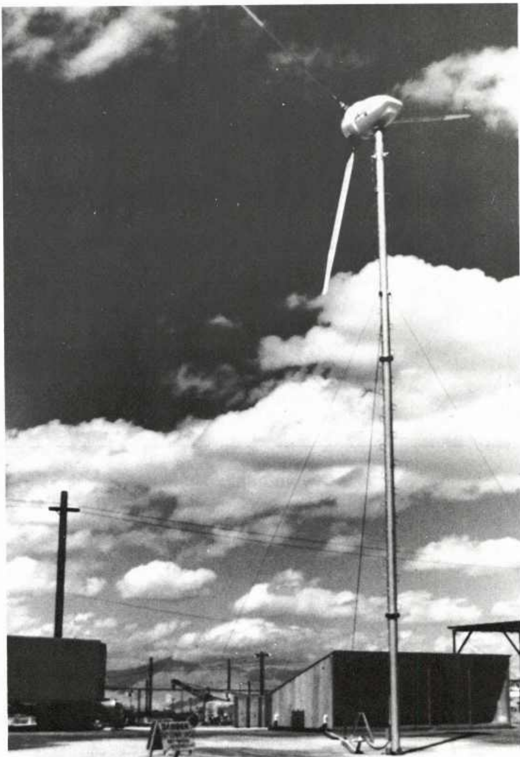
Figure 15. 9-kW WECS installed at NWC, China Lake.
