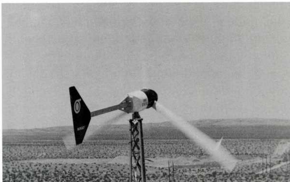
Figure 23. New 10-kW WECS installed at MCLB, Barstow.
