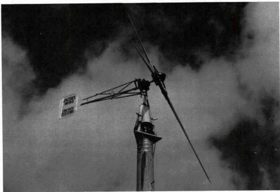
Figure 27. 12-kW WECS installed at Kaneohe Bay, Hawaii.
