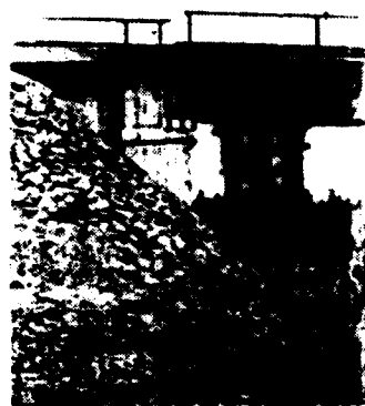
Fig. E24. The gap between the ends of the beam increased because of the tilt of the abutment.
