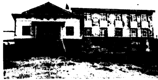
Fig. E42. Mangui railway station, which has a ventilated basement.
