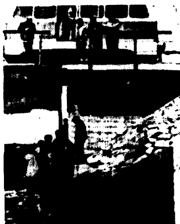
Fig. E24. The gap between the ends of the beam increased because of the tilt of the abutment.
