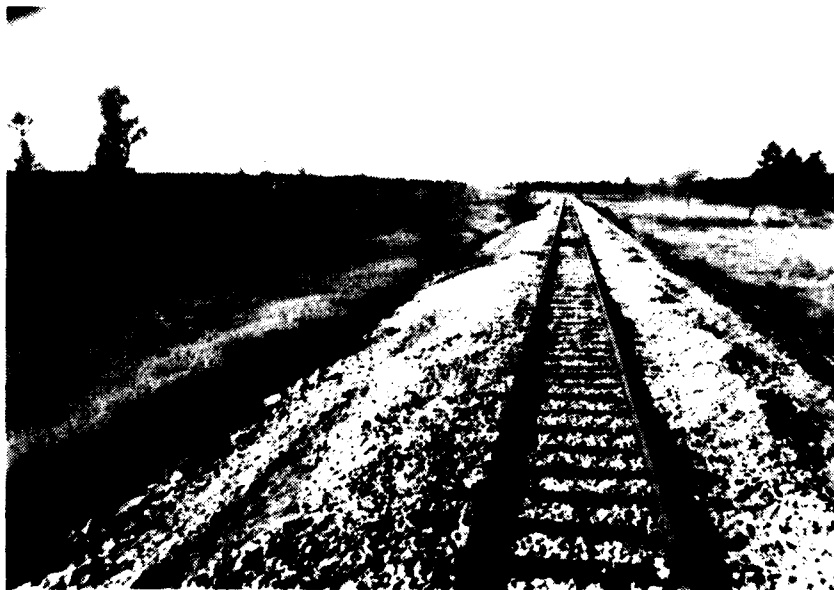
b. Characteristic roadbed in this area. Wood rail ties will be replaced with concrete ties. Drainage ditch is seen on left side. (Photograph by Ray A. Kreig.)
