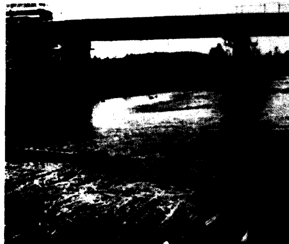
Figure 11. Stop 1. Steel plate girder bridge at 318 km on the Yalin Line. Access tubes in river and abutment are used to measure temperatures. Permafrost has been degrading under the riverbed. (See Figure 13 and text for details of bridge design and performance.)
