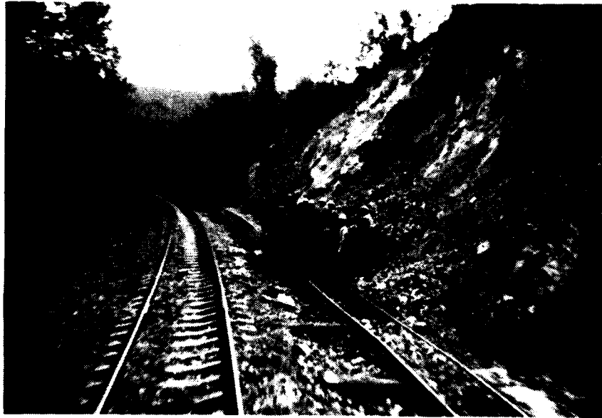
a. Widening of bedrock cut in Hsing An tunnel area. (Photograph by Ray A. Kreig.)
