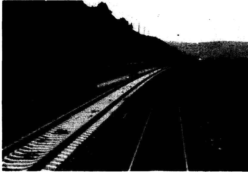
a. Double track with concrete ties. Retaining wall on left.
