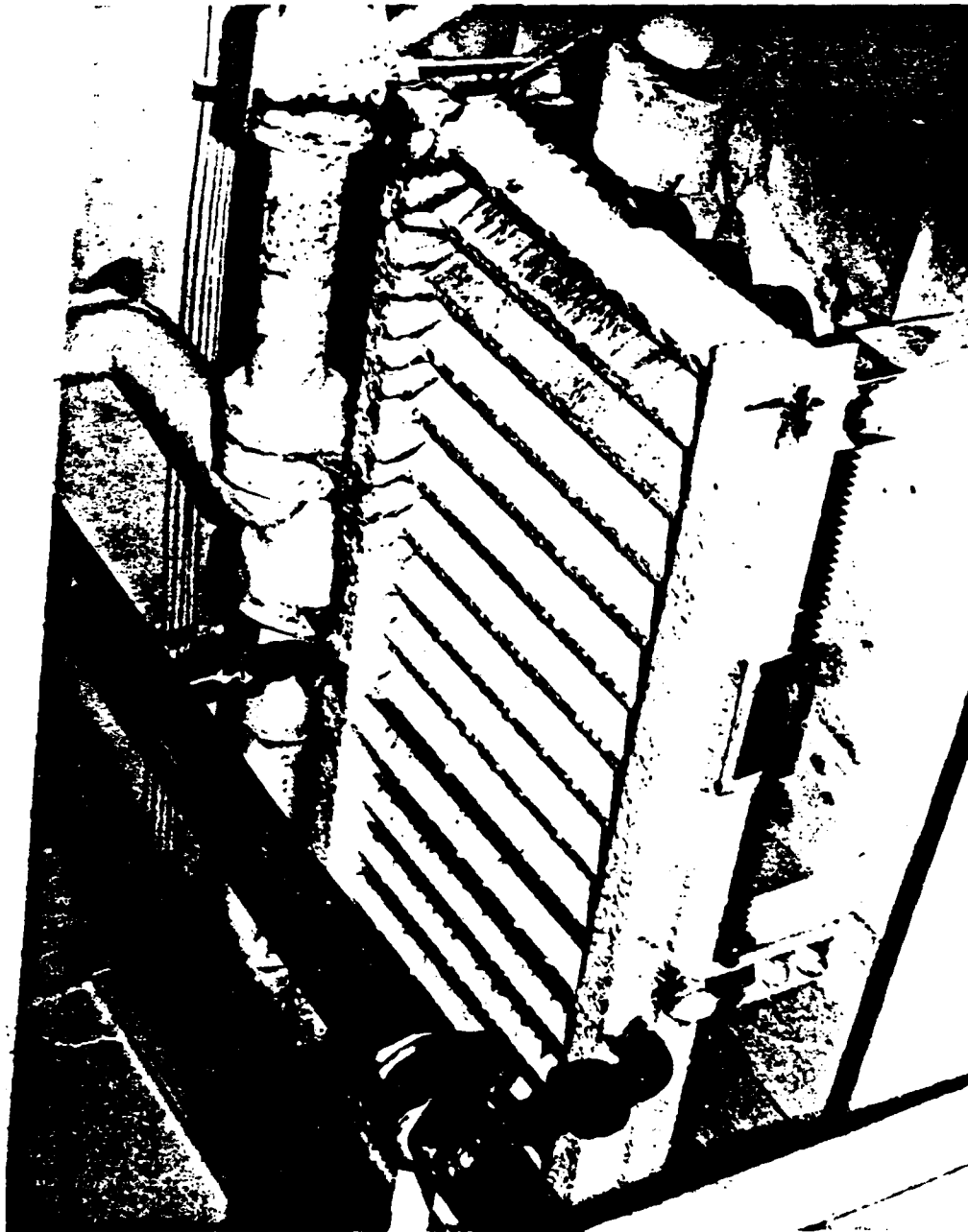
FIGURE 13. DAMAGED HEAT EXCHANGER IN CIWS MOUNT 21 MAGAZINE. BROKEN WELDS WHERE THE TANK IS ATTACHED TO THE MOUNTING BRACKETS CAUSED FLOODING OF THE MAGAZINE.
