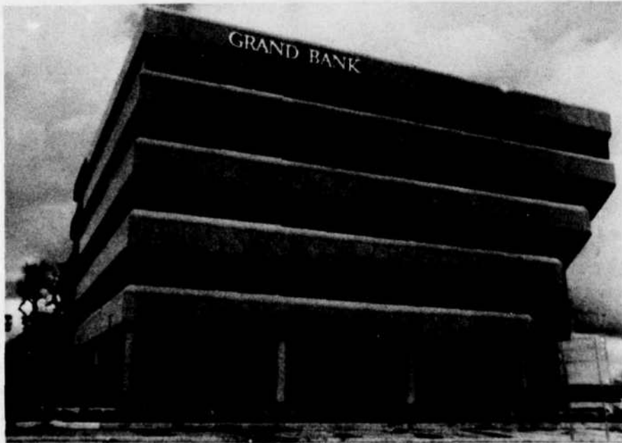
Figure 14. GFRC use on a bank building in Dallas, TX.
