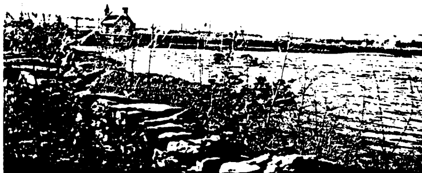
#77 DIAMOND HILL RESERVOIR - FROM EAST SIDE OF RESERVOIR LOOKING SW AT LONG EARTH EMBANKMENT TOPPED WITH CONCRETE WALL AND WITH RIP RAP ON POND SIDE 12/4/47
