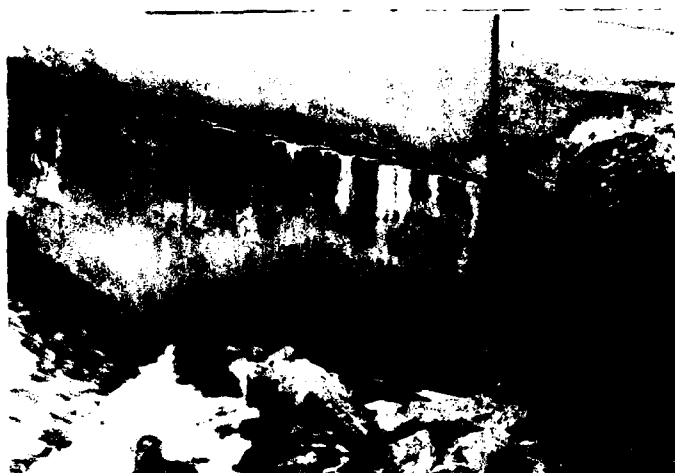
C-8 SEEPAGE AT COLD JOINT IN LEFT TRAINING WALL OF SPILLWAY
