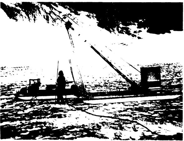
Figure 7. USGS Drill Sleds, South Cascade Glacier. Hose reel, winch drive, and boom sled in the foreground. Sled behind carries (right to left) the drill tank, electrically driven, high-pressure pump, water heater, and fuel tank. Operator is installing a hose spacer. Hose in the foreground brings water from a firm well near the previously drilled hole. Sleds are transported with a small track vehicle.
