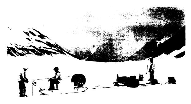
Figure 6. The Cal Tech sleds on Variegated Glacier, Alaska. Portable generator at the right, 55-gal fuel drum for the heater in the foreground. Gasoline engine-driven pump is behind the drum, between the tank and the heater. Hose reel, drive unit on the left sled. Operator on the far left is tending a cable to a pressure transducer down the same hole.
