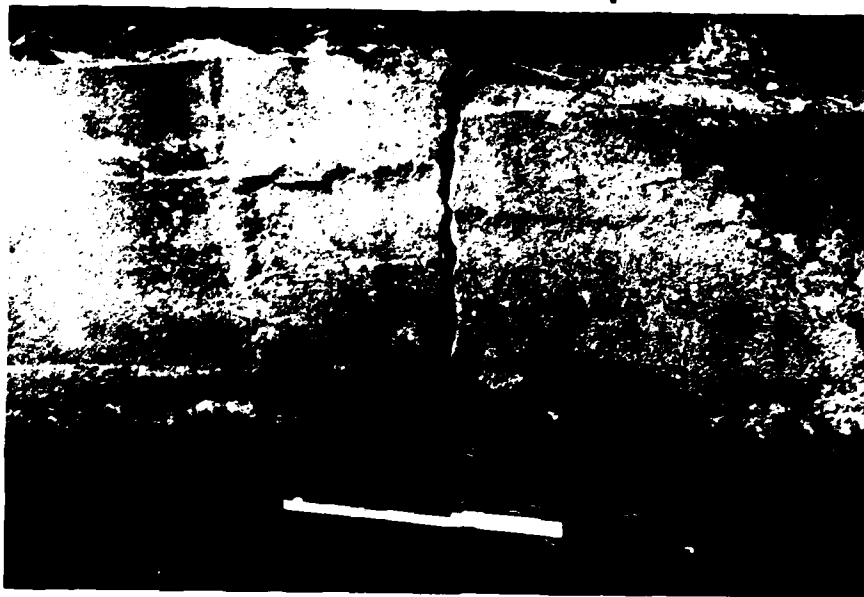
#1 CRACK AND MISALIGNMENT IN RIGHT WALL AND SLAB OF FLUME
