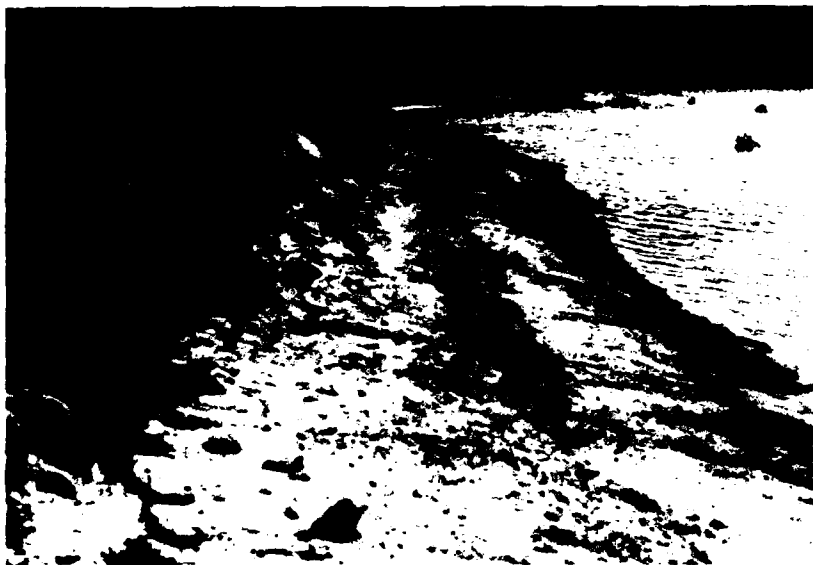
Photo 9. Upstream slope of dam. Slope measured approximately 1V:5H. Soil is slightly gravelly sand with some boulders.
