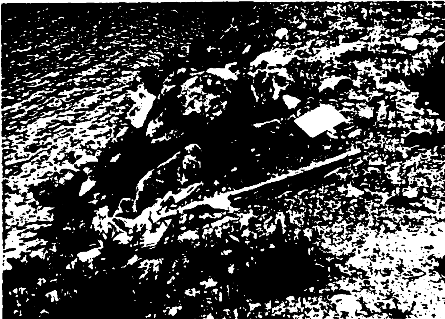
Figure 3 - Closeup of random fill placed on the upstream slope north of the outlet showing inadequacy of vegetative cover to prevent erosion.
