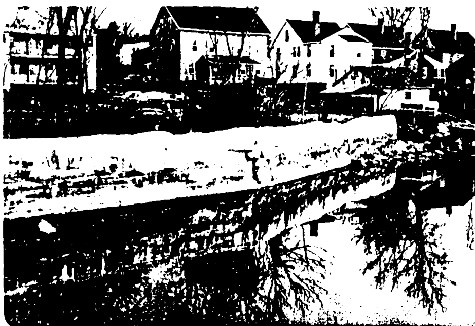
9. View from sluice gate structure showing deterioration of right upstream training wall
