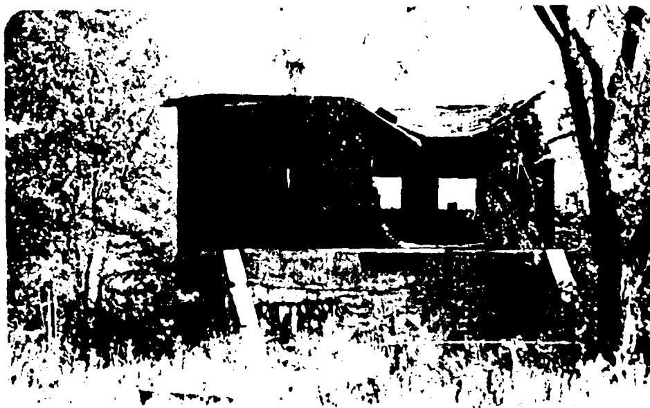
11. View from diversion channel showing deterioration of gatehouse
