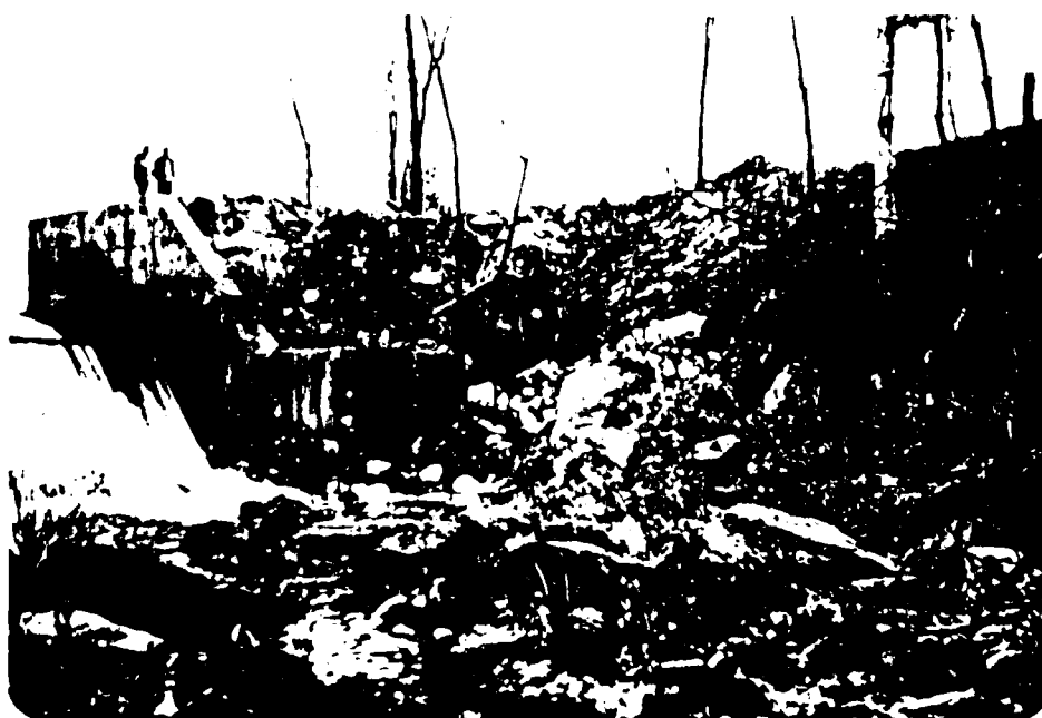
3. View from downstream channel of erosion and uncontrolled dumping at left abutment
