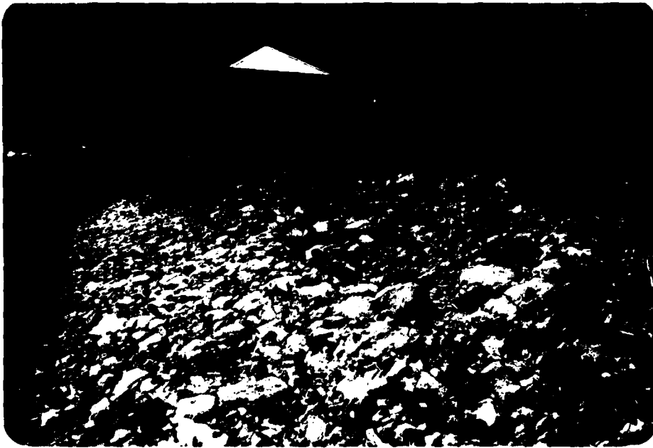
1. View from right abutment showing slope protection on upstream side of dam
