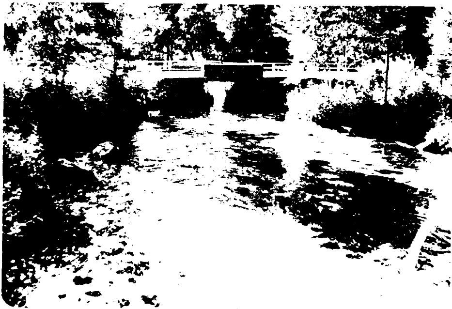
6. View of road bridge downstream of dam creating hydraulic constriction
