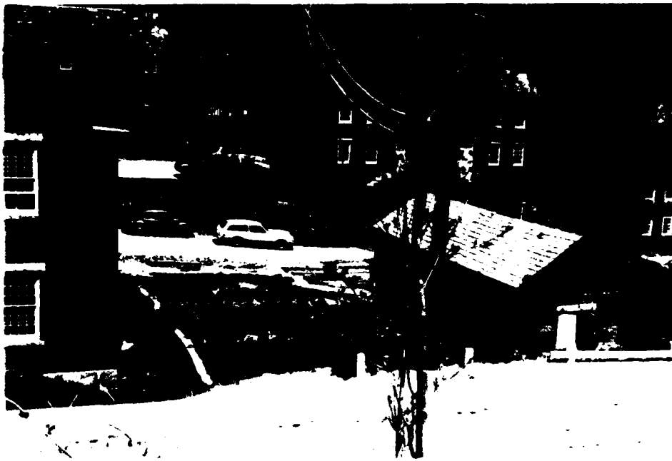
13. Upper Mill (Over the Dam) and the Toy Shop (Right). Downstream Channel Below These Buildings.
