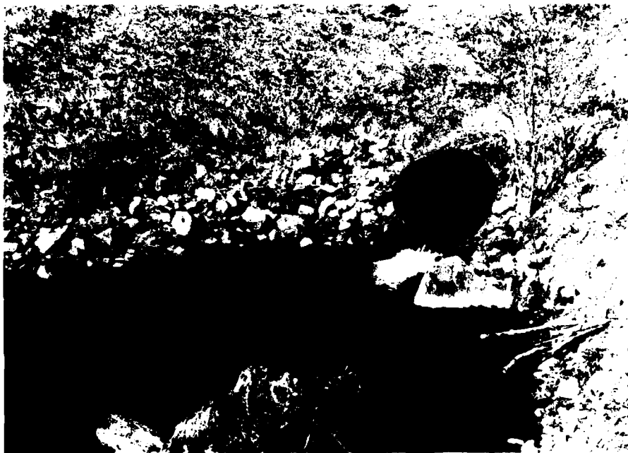
Figure 5 - View of 48" diameter discharge pipe. Note placed riprap at outlet.
