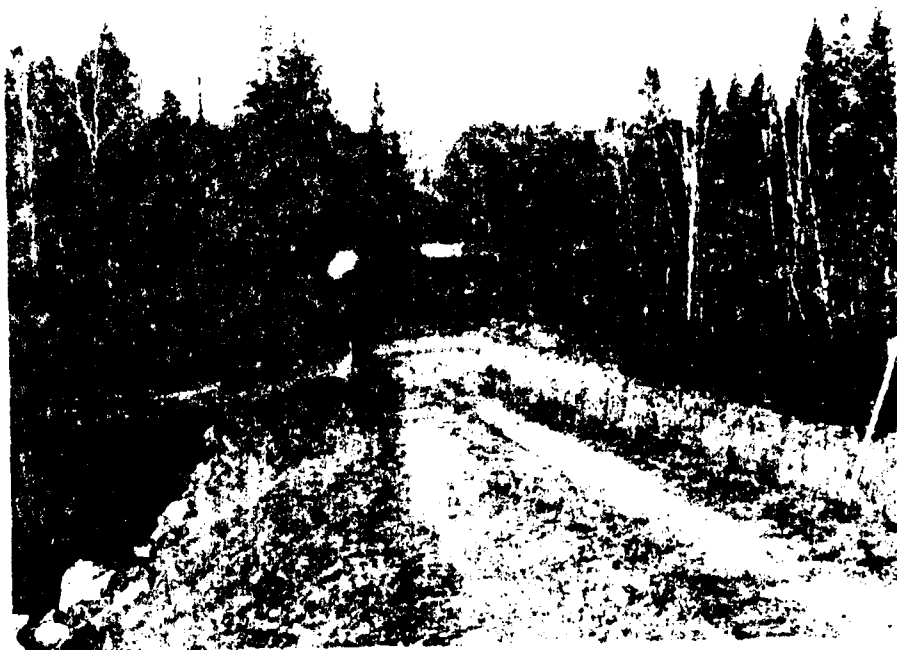
43. View of road leading to the site.
