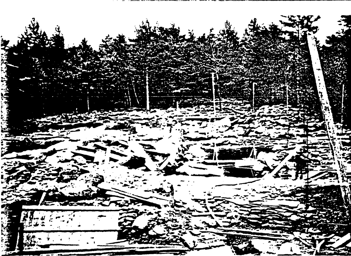
No. 1. Bennington Dam. Taken from the southerly bank of the river, looking northerly along proposed crest line of dam. July 1, 1924. 10:50 A.M.
