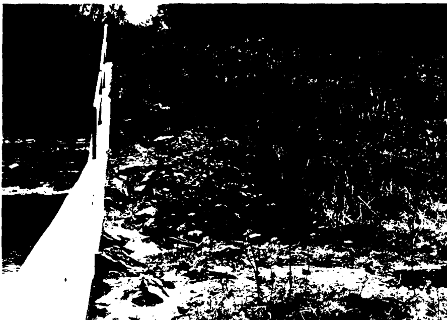
PHOTO NO. 17 - Erosion adjacent to the right side of the spillway.
