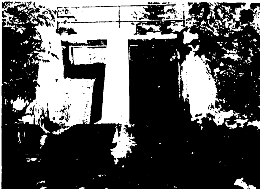
July 9, 1980 Photo 11 - View of the 2 concrete stoplog spillway bays from the downstream channel.
